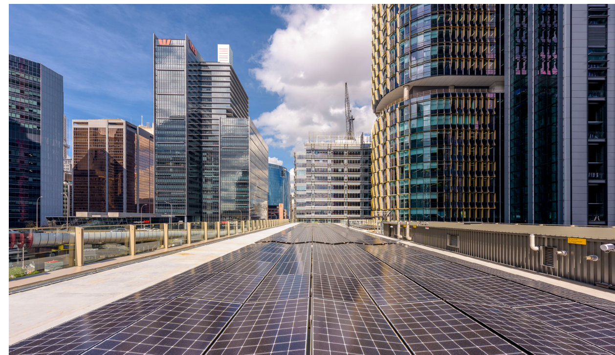
Rooftop Mounted Photovoltaic Array_Precedent Commercial Building C2
