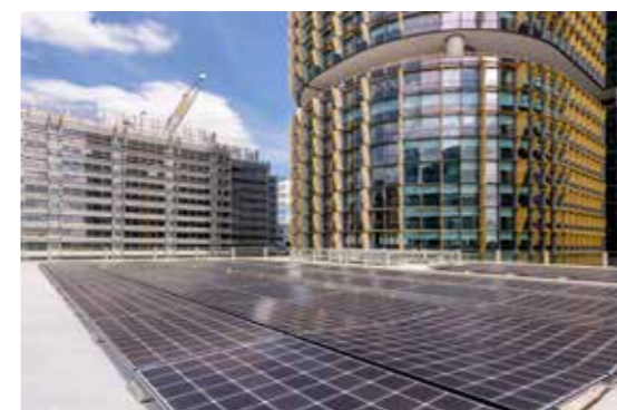
Photo voltaic Panels to Generate Renewable Energy
