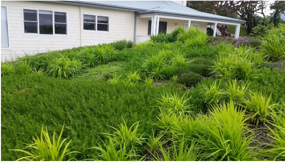
Residential green roof - Newport
