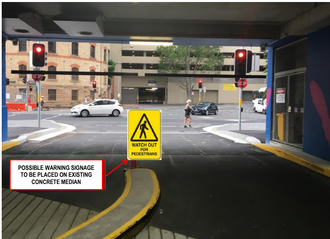
Figure 1-3 View of basement exit ramp (facing east) approaching the signalised intersection
