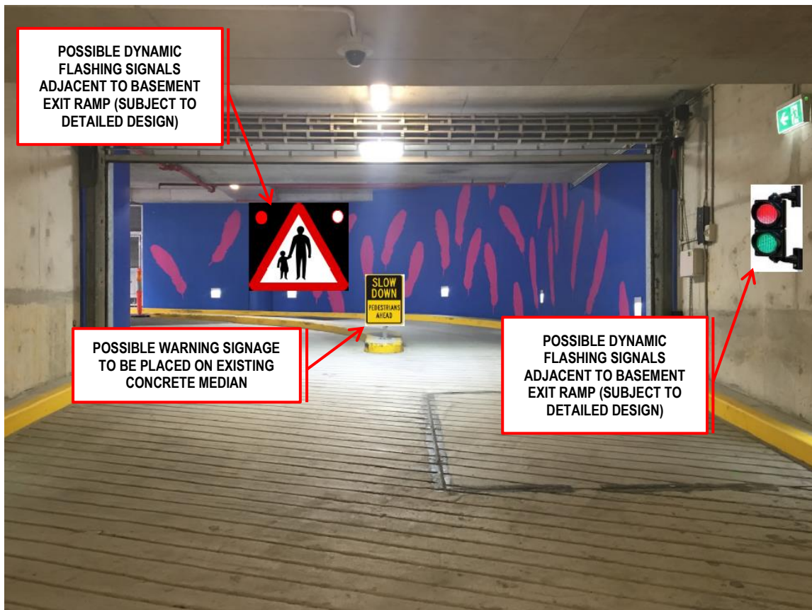
Figure 1-2 View of basement exit ramp (facing south) approaching the signalised intersection
