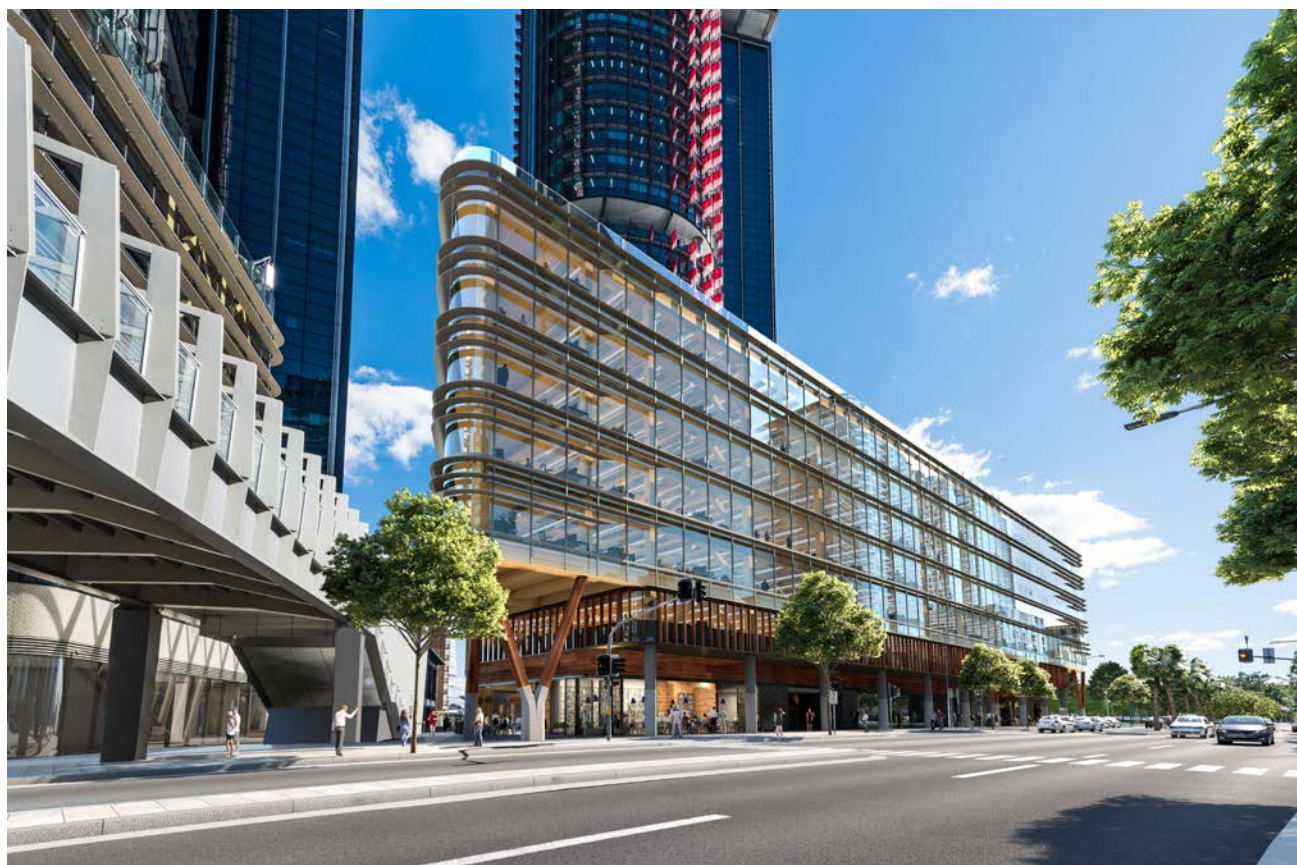
Figure 10 – Commercial Building C1 viewed from the south on Hickson Road
