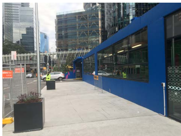
Existing basement exit on Hickson Road
