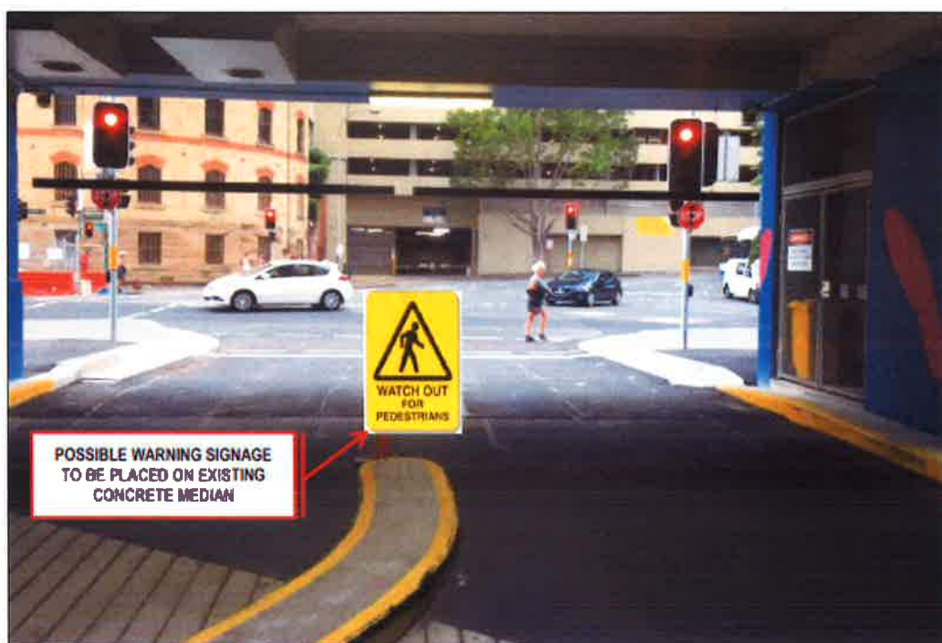
Figure 12: View of basement exit ramp (facing east) approaching the signalised intersection (Applicants EIS)
