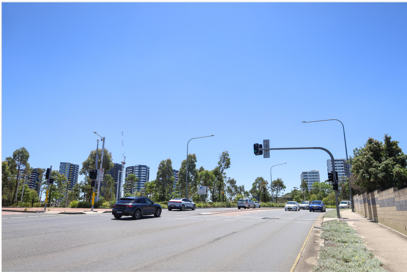
Existing site photo - Old Northern Road
