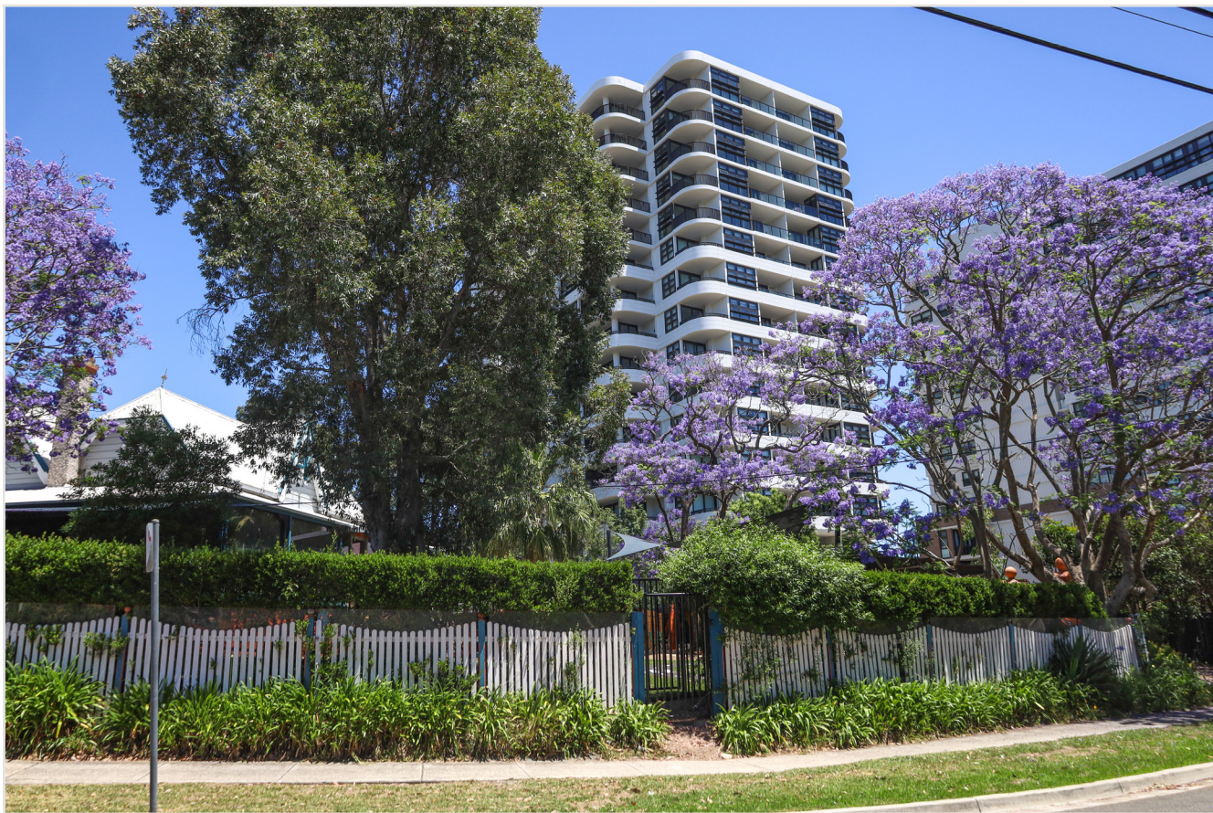
Existing site photo - Garthowen Cres
