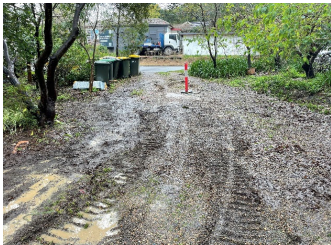
View of driveway into No. 20 Looking north Inspected 22.08.2025
