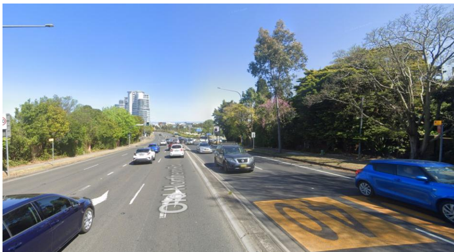
Figure 2-8: Old Northern Road (Facing Westbound)
