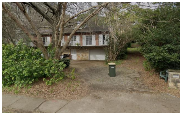
Figure 5 20 Old Castle Hill Road and shared driveway to 18 Old Castle Hill Road
