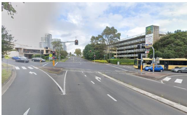
Figure 12 Intersection of Old Castle Hill Road, McMullen Avenue and Pennant Street; Castle Towers car-park to the right
