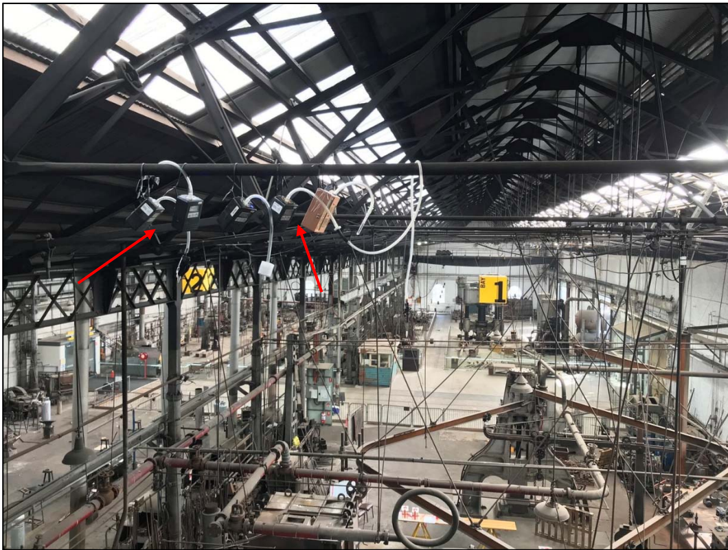
Photograph 3: Air sampling was conducted at 1.5 metres and truss height at each location.
