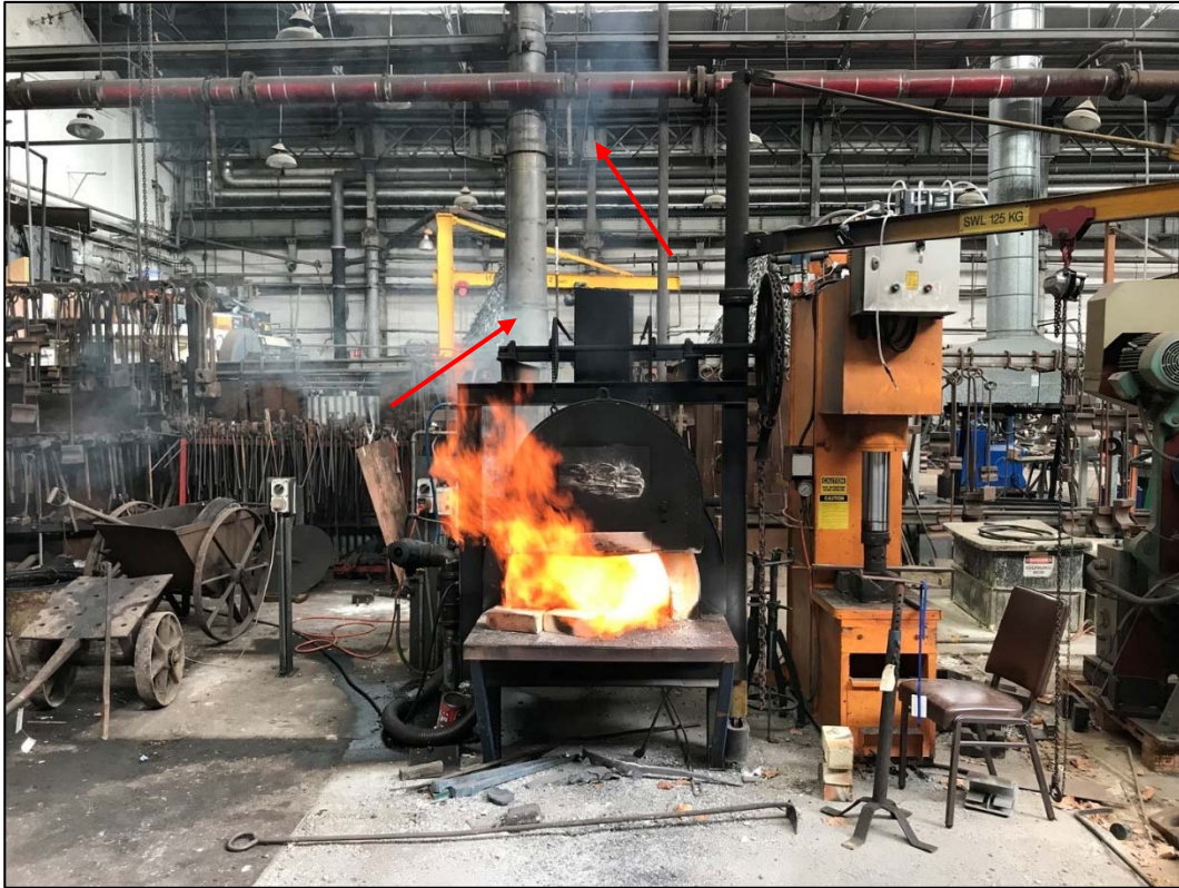
Photograph 1: Visible smoke and fume generation following start-up of the Big Major Oil Furnace, accumulates beneath the roof apex and slowly releases to atmosphere via the roof louvres.
