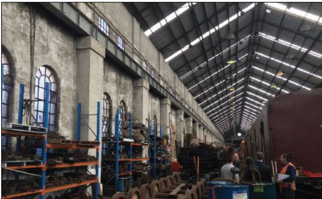
Figure 6.1: Roof profile of the Large Erecting Shed (Source: Ethos Urban)
