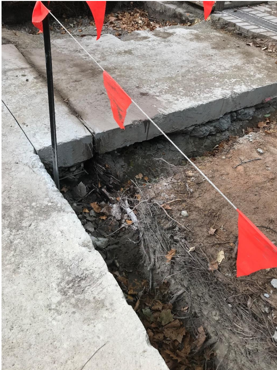
Figure 3: Existing reinforced concrete slab on grade
