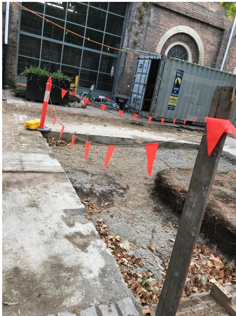
Figure 2: Existing reinforced concrete slab on grade
