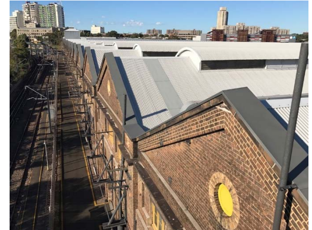
Photo 3: Locomotive Workshop – North aspect, looking east
