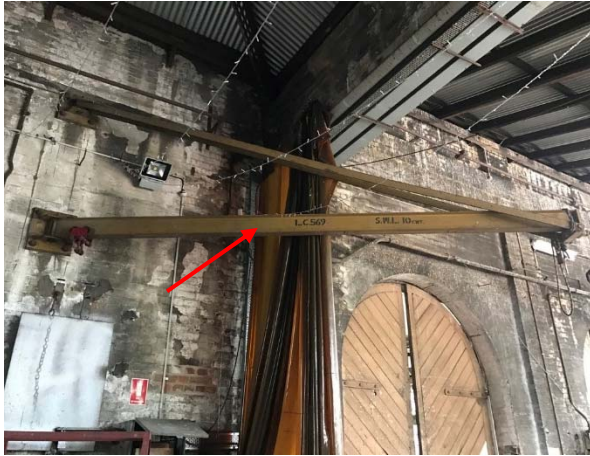
Photo 13: Exterior – SE Annex, XRF screening of the grey and yellow jib cranes identified lead based paint
