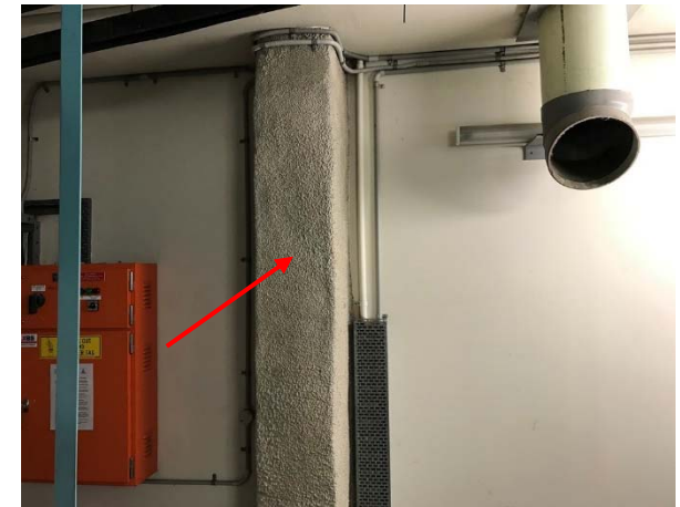
Photo 48: Bay 3 north - The vermiculite fire-rating insulation in the northern Level 2 plant room does not contain asbestos
