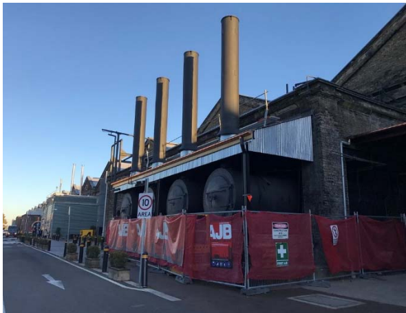
Photo 4: Exterior – Boiler House
