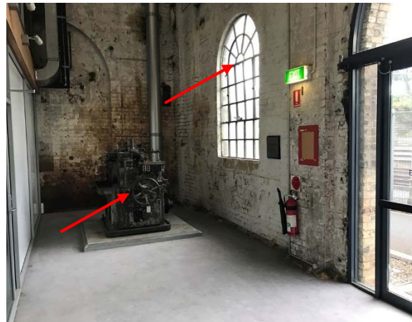
Photo 95: Bay 15 – Analysis and XRF screening of off-white arched heritage window frame on the northern wall and the majority of heritage machinery on display throughout the bay identified lead based paints
