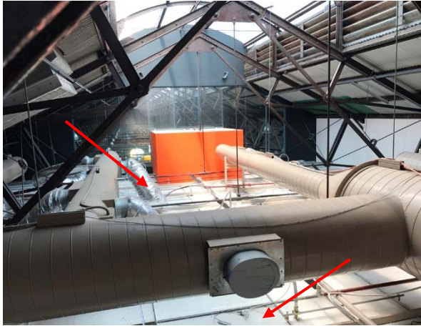
Photo 55: Bay 4 north – Fixed and flexible air-conditioning ductwork within office ceiling cavities is insulated with SMF. Lead impacted settled dusts may be present on the ductwork and ceiling tiles in Level 2 ceiling locations that are directly below exposed roof trusses.
