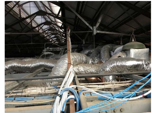
Photo 102: Bay 16 – Lead dust samples collected from the flat roofs of the northern and southern office blocks identified lead contaminated dusts. Fixed and flexible air-conditioning ductwork on the Level 1 office roof is insulated with SMF.
