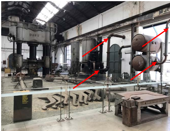
Photo 28: Bay 1 - Non-rubberised gaskets associated with the old steam plant throughout Bays 1 and 2 are suspected to contain asbestos
