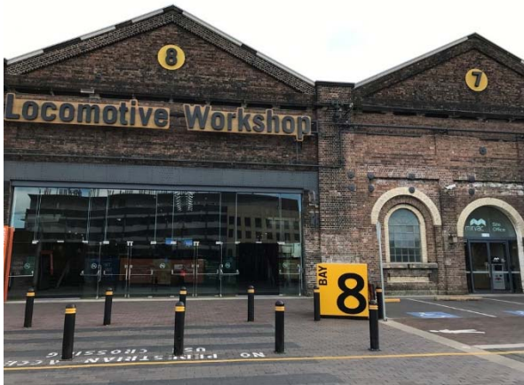
Photo 1: Locomotive Workshop – 2 Locomotive St, Eveleigh
