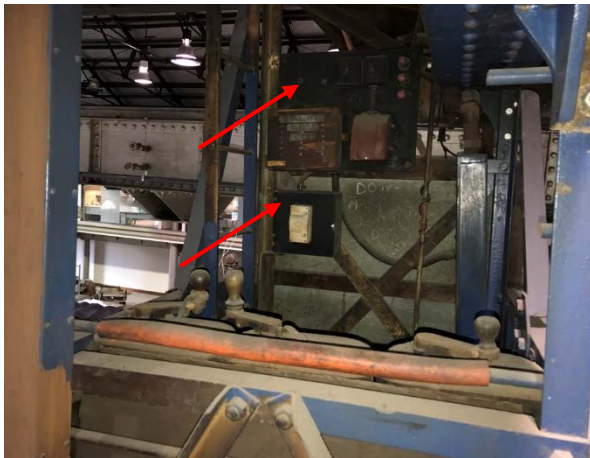
Photo 82: Bays 10 - 14 - Black electrical boards in the operators cabins of the overhead travelling cranes are presumed to contain asbestos
