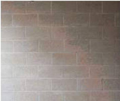
Concrete block to new solid intertenancy walls
