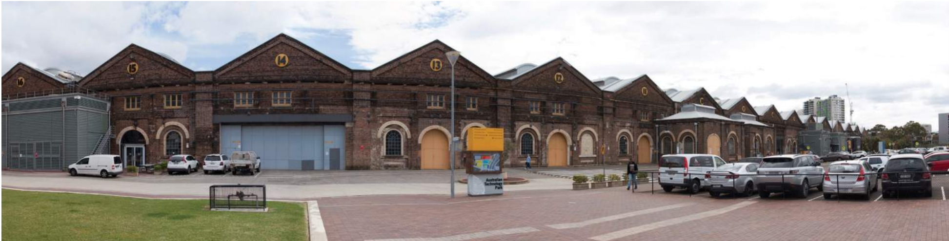
Panoramic view of south elevation along Locomotive Street
