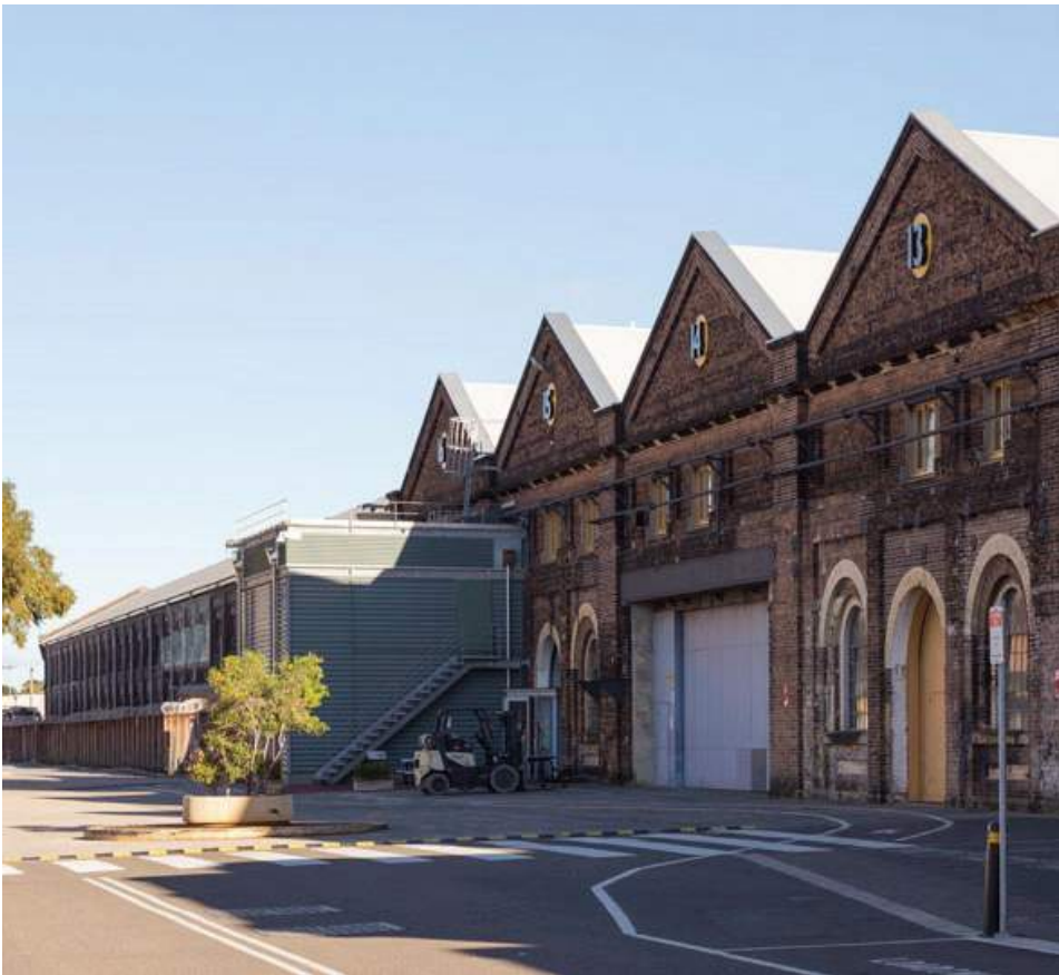
View of substations looking west down Locomotive Street
