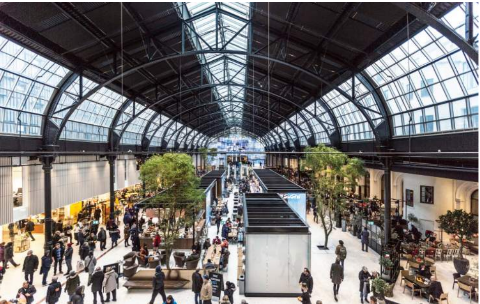
Exposed wrought ironwork at Ostbanenhallen, Oslo
