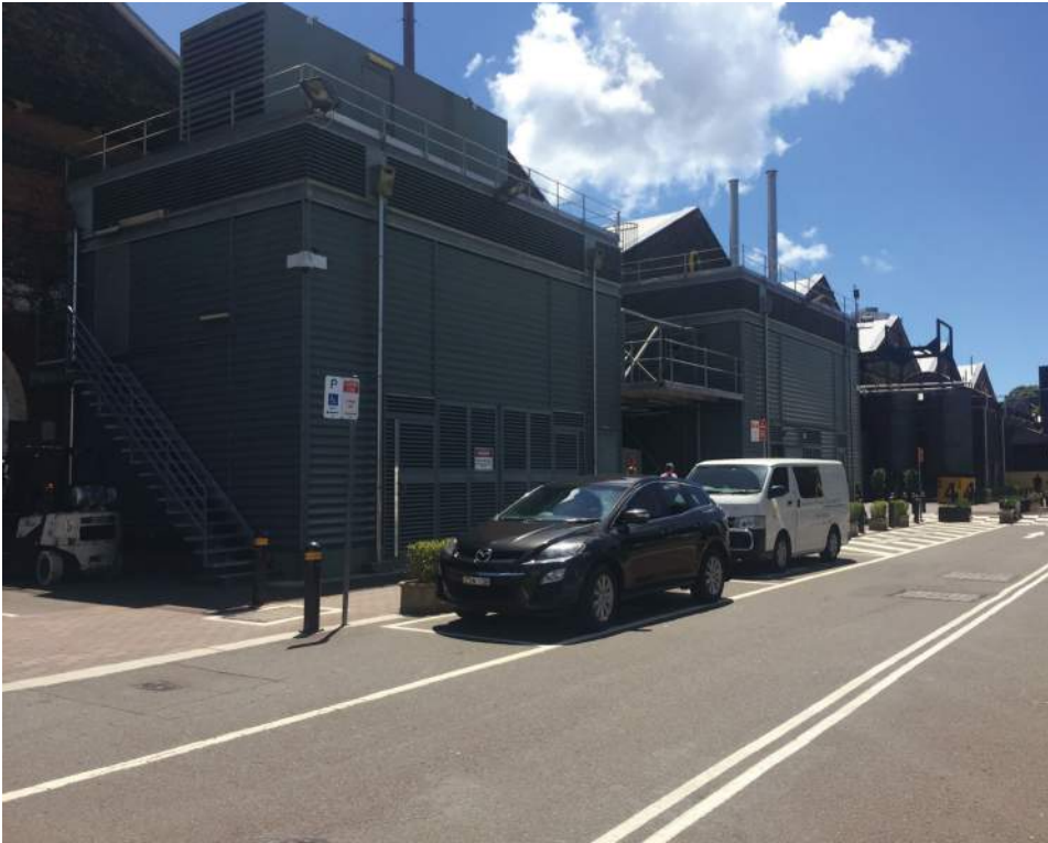
Substations on the southern facade
