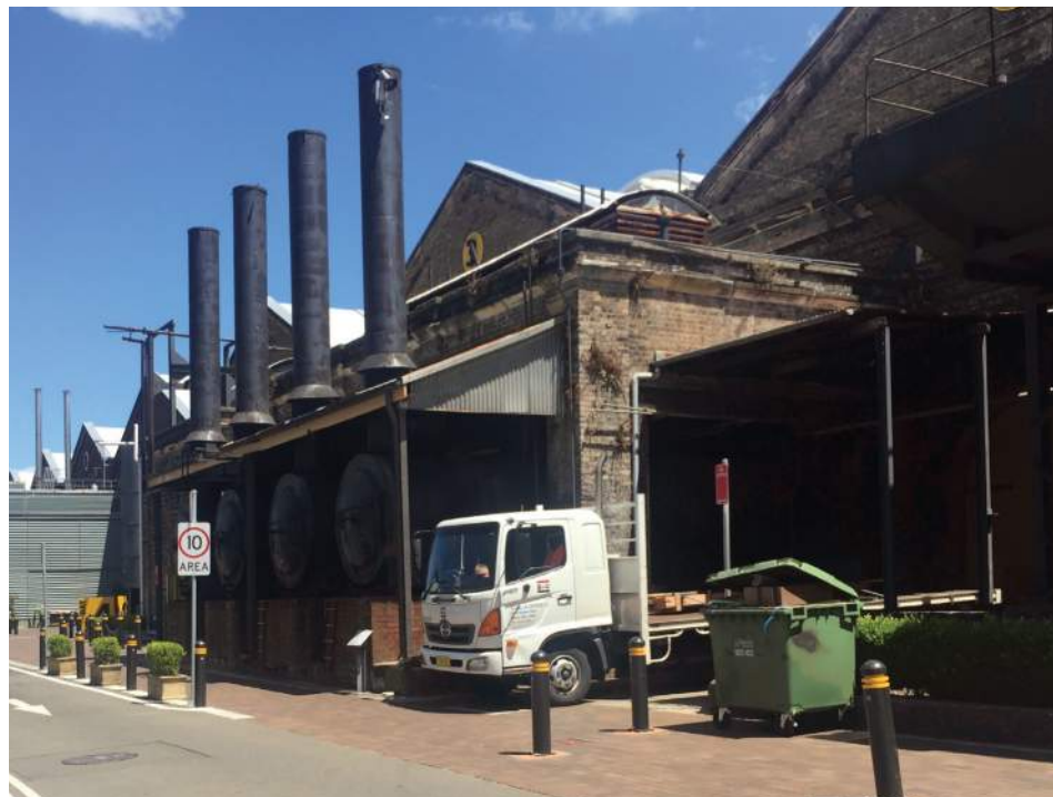
Existing exterior heritage conditions
