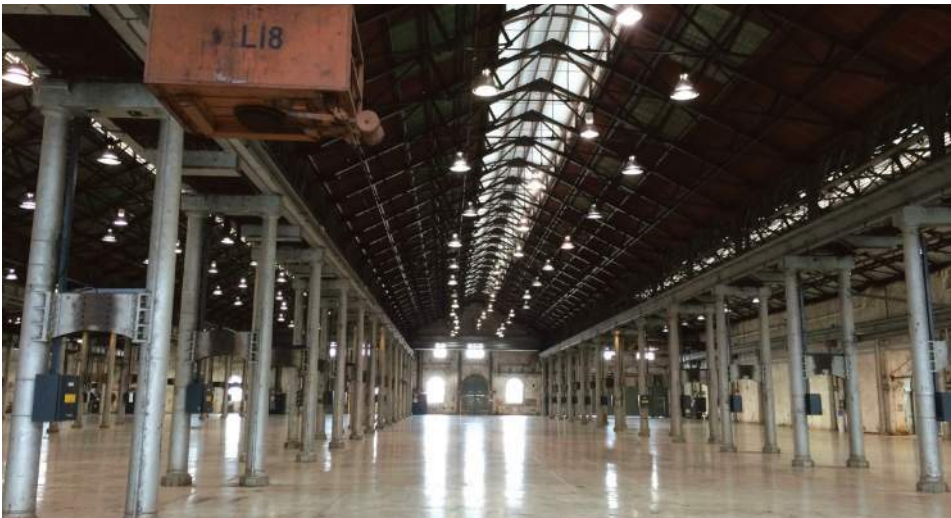
Exhibition hall looking toward south elevation
