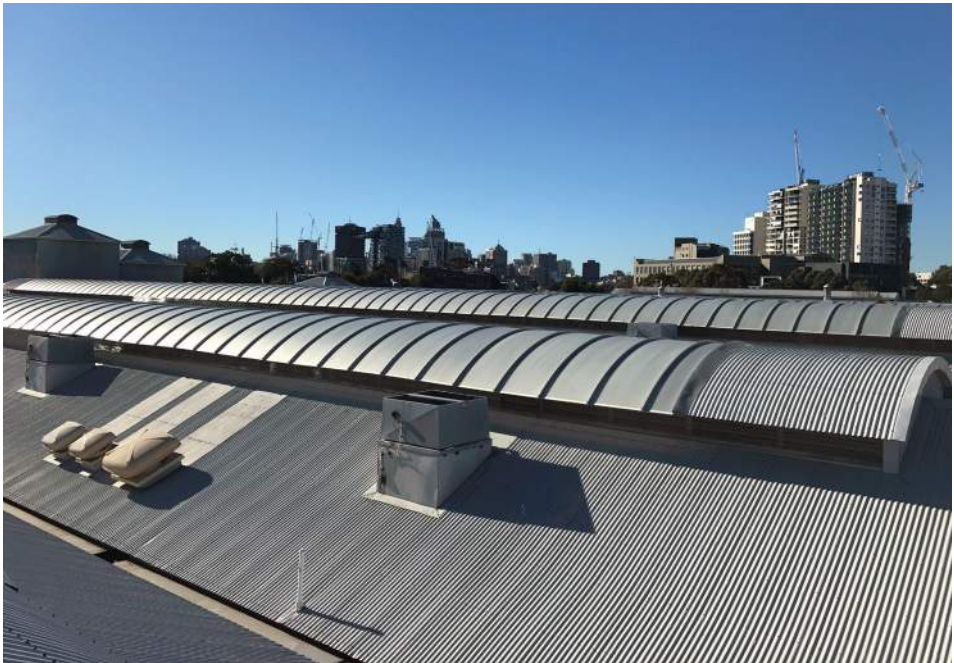
Existing roof conditions
