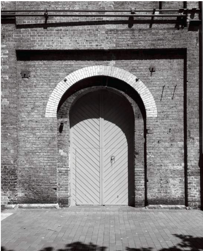
Arched heritage opening on southern facade
