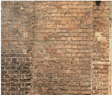
Existing heritage brick facade retained
