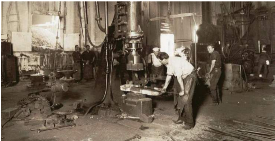
Metal forging on the steam hammer, 1926
