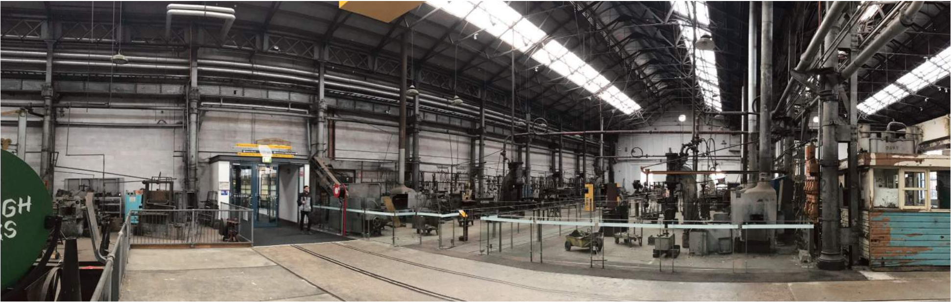
Existing intertenancy wall between bays 2 and 3 - modern infill block work
