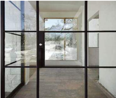
Glass infill to new external openings
