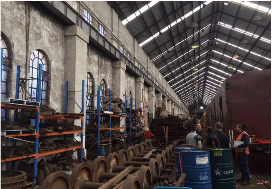
Existing roof conditions at the Large Erecting Shed, adjacent to the site
