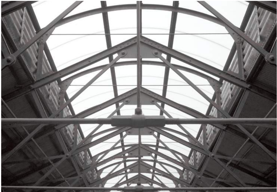
Heritage truss detail with existing polycarbonate roof
