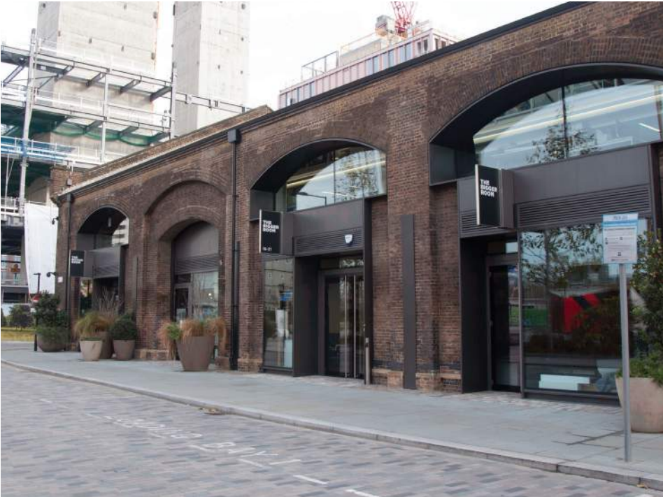
Treatment to heritage openings at Kings Cross Station, London
