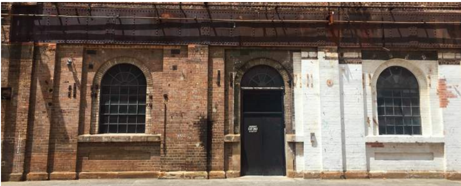
Heritage openings at Carriageworks
