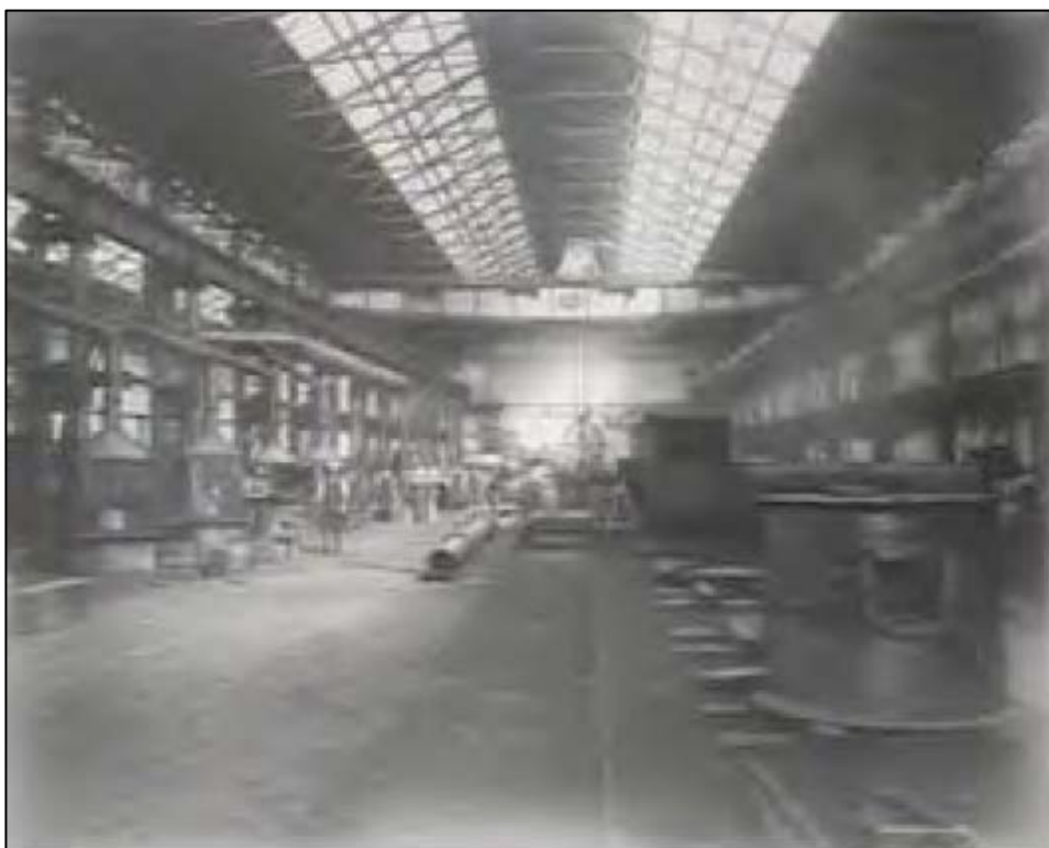
FIGURE 5: INTERIOR OF THE LOCOMOTIVE WORKSHOPS, DATE UNKNOWN. (SOURCE: GOVERNMENT PRINTING OFFICE COLLECTION, STATE LIBRARY OF NSW)
