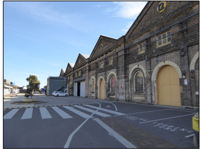
FIGURE 10: FRONT FAÇADE OF LOCOMOTIVE WORKSHOP, BAYS 12 TO 16 (SOURCE: CURIO 2016)
