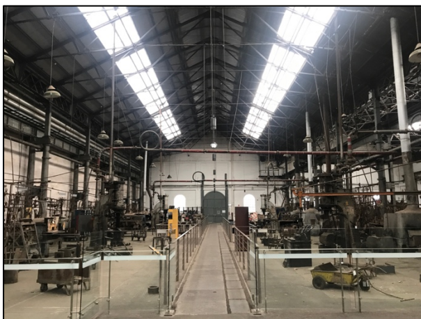
FIGURE 11: ROOF IN BAY 2, SOUTH. (SOURCE: ETHOS URBAN 2016)
