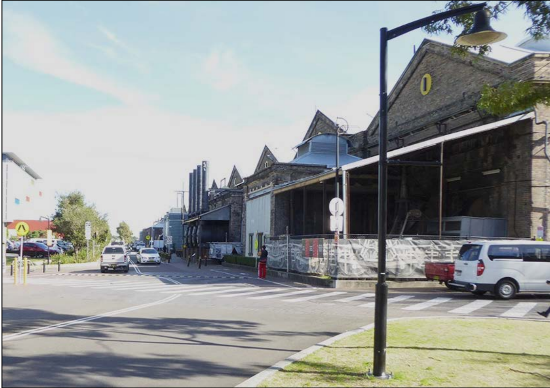
FIGURE 90: EXISTING 'LEAN-TO' AND ATTACHED BRICK ANNEX ON SOUTHEAST CORNER OF BAY 1, VIEW WEST ALONG LOCOMOTIVE STREET (SOURCE: CURIO 2016)
