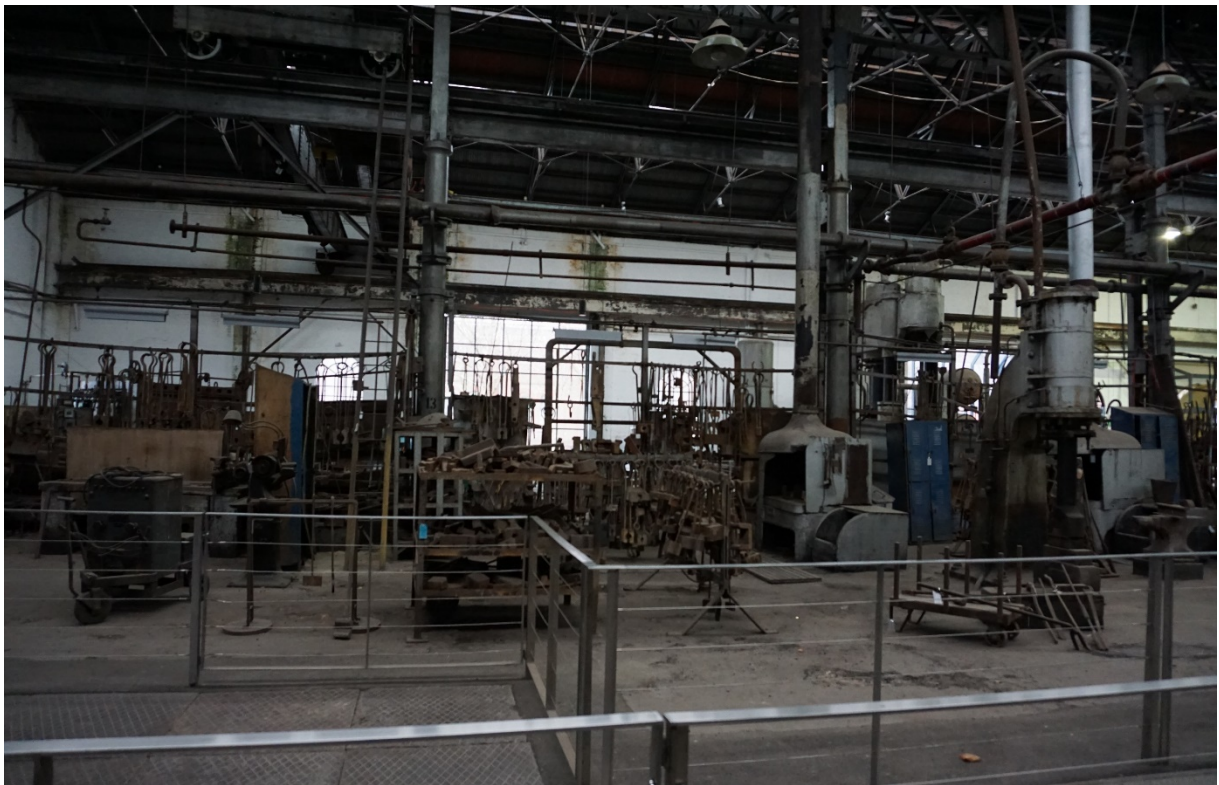
FIGURE 53: EXISTING CROWDED, STATIC MOVEABLE HERITAGE DISPLAY IN BAYS 1 & 2 NORTH. MANY ITEMS NOT INSITU (SOURCE: CURIO 2016)
