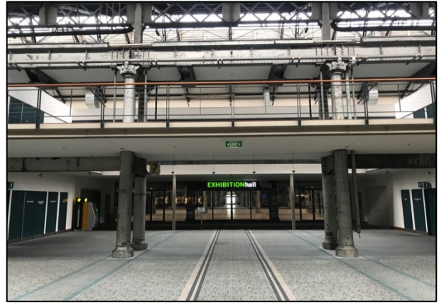
FIGURE 20: MEZZANINE LEVEL ACROSS BAY 9 [NOW BAY 8], VIEW WEST TO ENTRANCE TO EXHIBITION HALL IN BAYS 10–14 [NOW BAYS 8–13] (SOURCE: ETHOS URBAN 2016)
