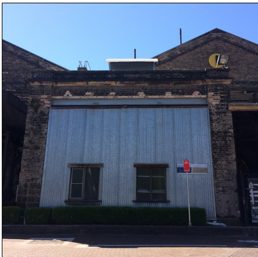
FIGURE 89: EXISTING BAY 1 BRICK ANNEXE ADJACENT TO 'LEAN-TO' (SOURCE: CURIO 2016)
