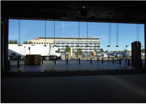
FIGURE 19: GLASS OPENING AT SOUTHERN END OF BAY 8 [NOW BAY 7] (SOURCE: CURIO 2016)
