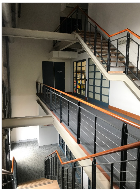
FIGURE 67: BAY 3 NORTH, FACING EAST, EXISTING TWO STOREY OFFICE FIT-OUT, MODERN FABRIC EASTERN INTERTENANCY WALL, PROPOSED FOR DEMOLITION (SOURCE: ETHOS URBAN 2017)
