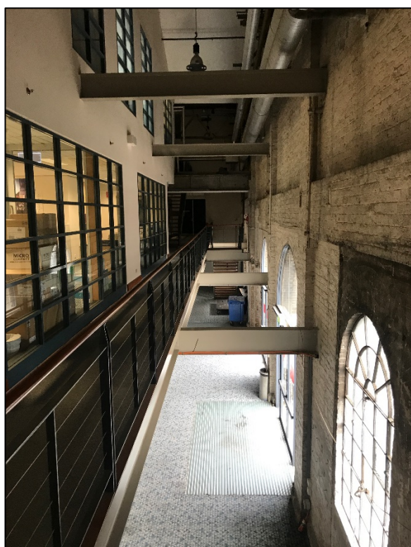
FIGURE 66: EXISTING OFFICE FIT-OUT, MEZZANINE FIRST STOREY, ATTACHMENT TO NORTHERN WALL, BAY 3 NORTH (SOURCE: ETHOS URBAN 2017)
