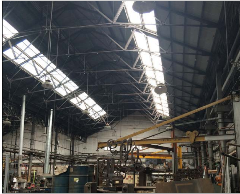
FIGURE 82: EXISTING ROOF IN BAYS 1 AND 2 (SOURCE: CURIO 2016)
