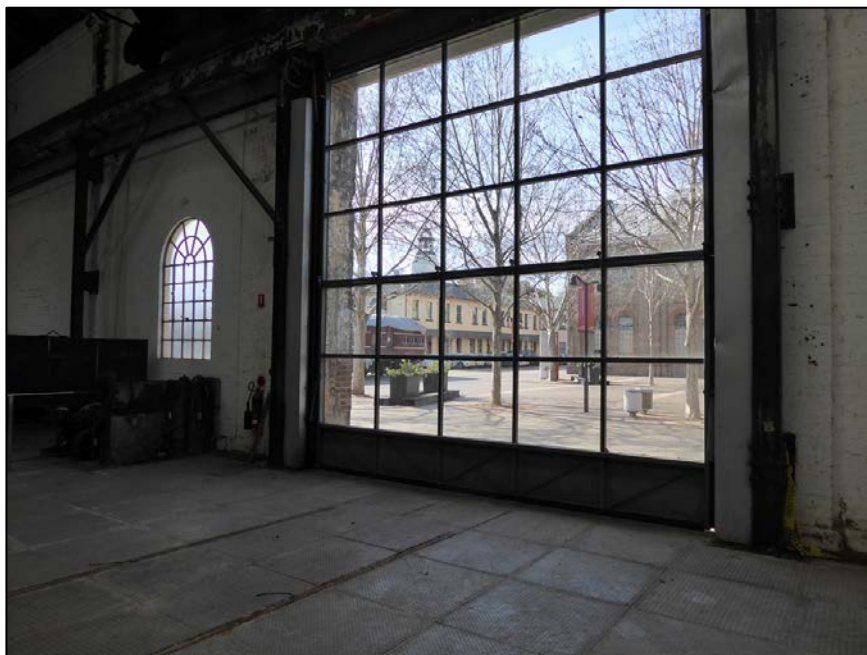
FIGURE 87: EXISTING LARGE FORMAT GLASS PANELLED ROLLER DOOR IN NORTHEAST OF BAY 1, PROPOSED FOR REPLACEMENT (SOURCE: CURIO 2016)
