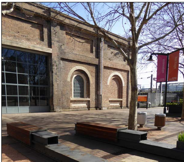
FIGURE 88: VIEW NORTHWEST ALONG EASTERN FAÇADE OF LOCOMOTIVE WORKSHOP FROM INNOVATION PLAZA, ROLLER DOOR PROPOSED FOR REPLACEMENT FOR LOADING DOCK ENTRANCE, AND NORTHEASTERN BRICKED OVER WINDOW PROPOSED FOR RESTORATION (SOURCE: CURIO 2016)
