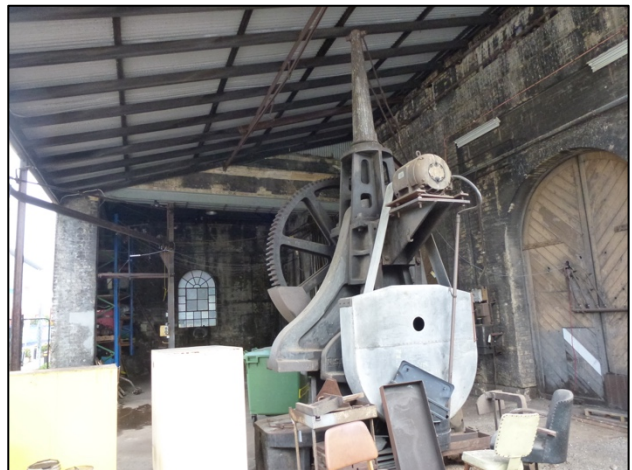
FIGURE 92: HERITAGE GUILLOTINE WITHIN EXISTING EXTERNAL 'LEAN-TO' ALONG SOUTHERN FAÇADE OF BAY 1 (SOURCE: ETHOS URBAN 2017)
