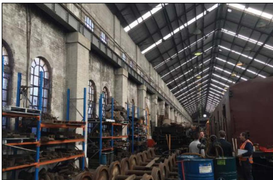
FIGURE 78: ROOF PROFILE OF THE LARGE ERECTING SHED (SOURCE: ETHOS URBAN)
