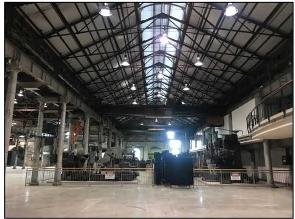
FIGURE 22: MACHINERY GROUPS IN NORTH OF BAY 10 [NOW BAY 9] (SOURCE: ETHOS URBAN 2016)
