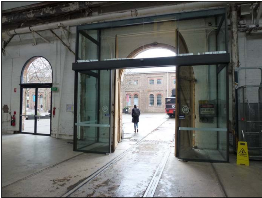
FIGURE 86: EXISTING CENTRAL TIMBER ENTRANCE DOORS IN BAY 1 FROM INNOVATION PLAZA, TO BE RETAINED IN FIXED OPEN POSITION N.B. CURRENT INTERNAL GLAZED PARTITION DOOR AS VISIBLE IN IMAGE TO BE REMOVED THROUGH PROPOSED DEVELOPMENT. (SOURCE: ETHOS URBAN 2017)
