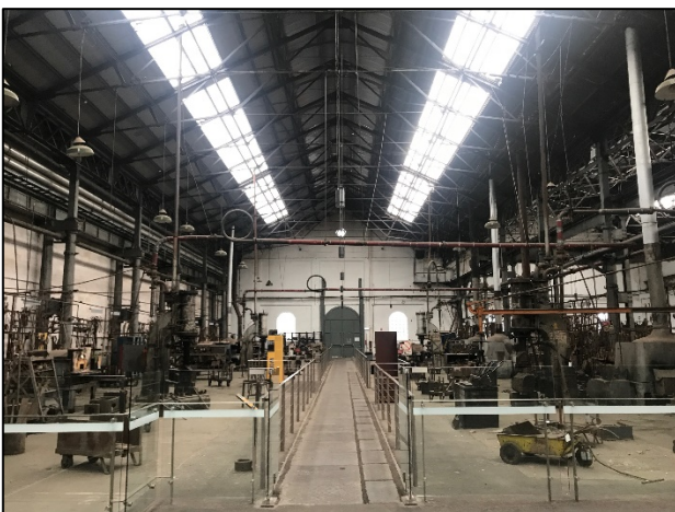
FIGURE 56: EXISTING INTERPRETATIVE ELEMENTS (GLASS BALASTRADES AND WIRE FENCING), BAY 1 NORTH, PROPOSED FOR DEMOLITION (SOURCE: ETHOS URBAN 2017)
