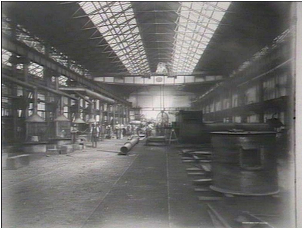
FIGURE 80: INTERIOR WORKSHOPS DURING ERW FUNCTION, VIEW TO HERITAGE TRUSSES AND ROOF SKYLIGHTS, DATE UNKNOWN (SOURCE: STATE LIBRARY OF NSW)
