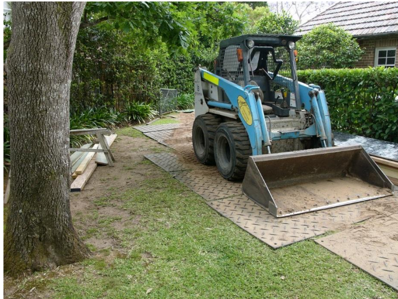
Figure 4 – Showing typical detail for truck mats.
