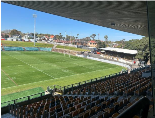
Figure 28: View of Leichhardt Oval showing seating bowl, grandstand and surrounding
