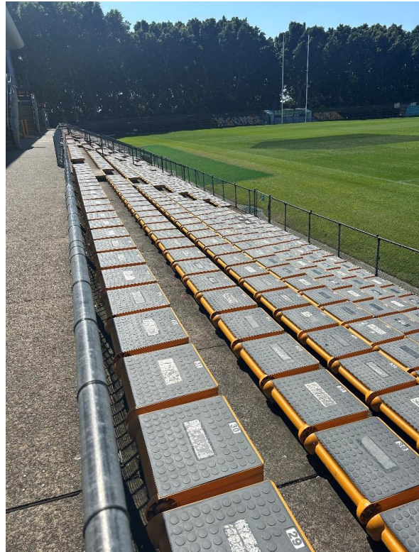
Figure 30: View of lower seating bowl on Western Grandstand
