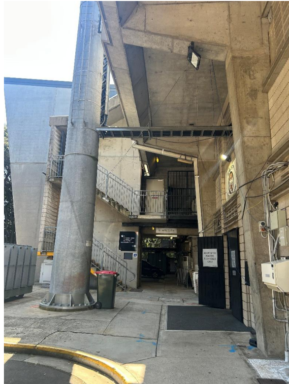
Figure 34: Western façade and stairway to mezzanine level
