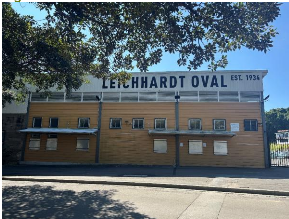
Figure 49: Keith Barnes Stand, looking north
