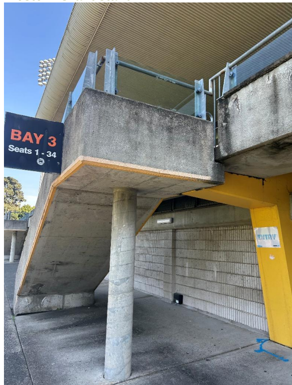
Figure 32: Access stairs to seats in Western Grandstand
