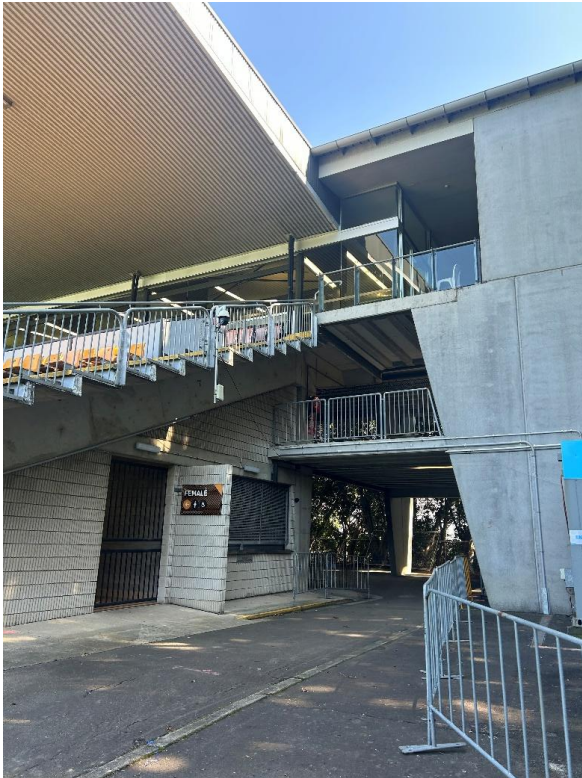
Figure 33: Northern façade and stairway to mezzanine level
