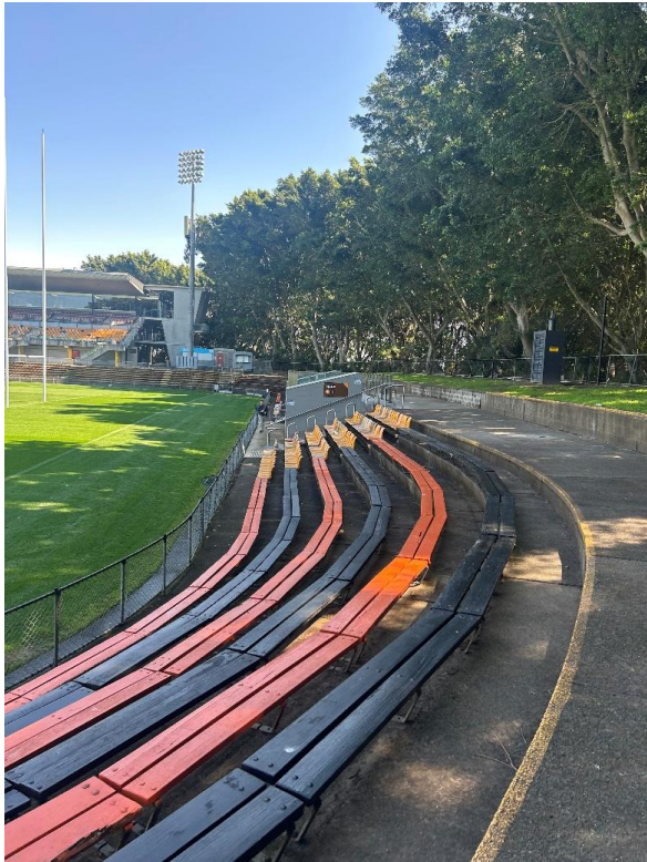
Figure 50: Northern end of Lower Seating Bowl, looking west
