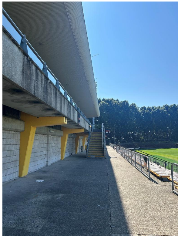
Figure 36: Eastern Façade, looking north
