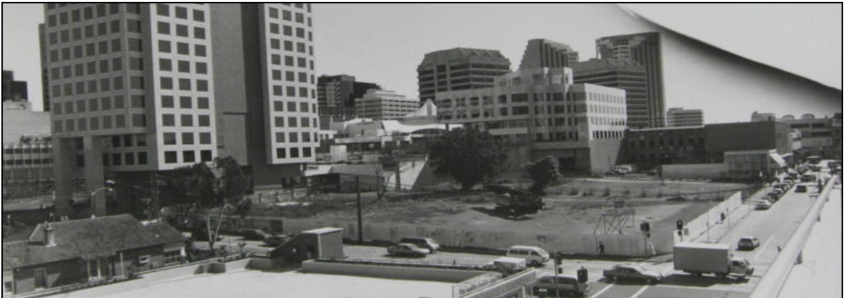
Figure 3-8: Photograph of the Mandarin Centre construction site, taken in 1993. (Source: Willoughby City Library)
