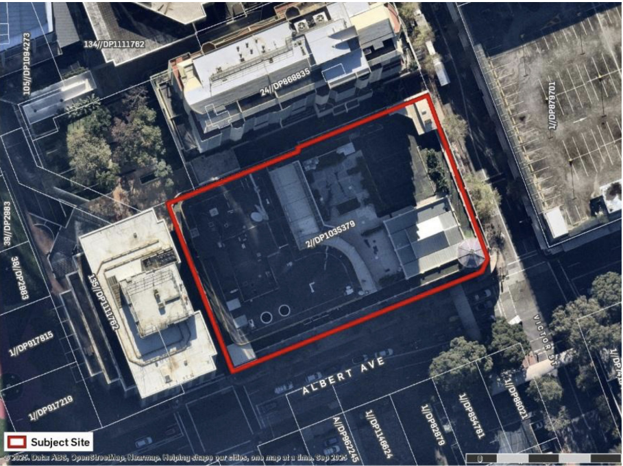
Figure 1.2 Aerial Photograph. Source:Urbis, 2025
