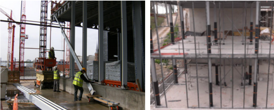
Figure 1.5 Typical Construction of Stick System
