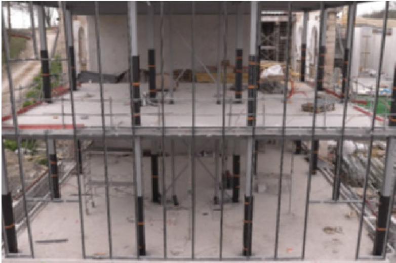
Figure 1.11 Typical Construction of Stick System
