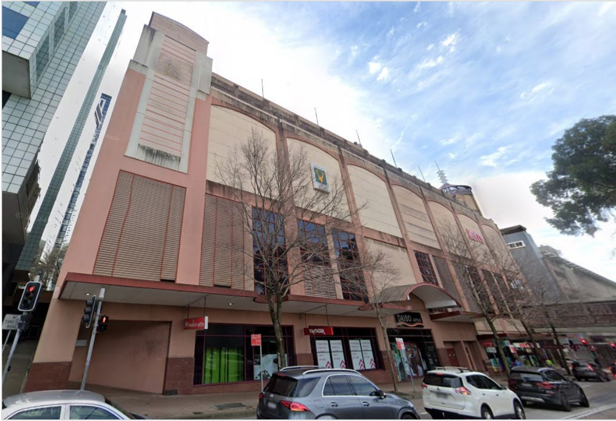
Figure 3-9: View of the south-facing elevation of the Mandarin Centre. (Source: Google. 2024)
