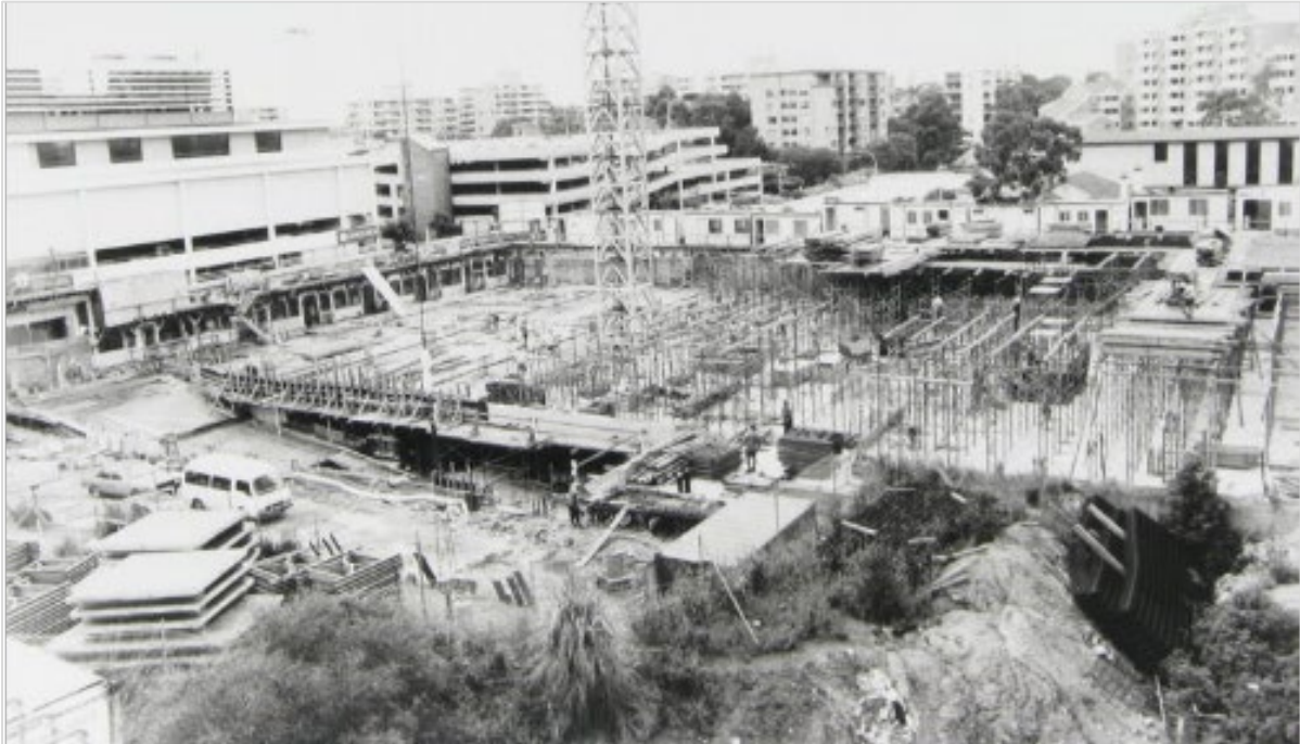
Figure 2-6: Photograph of the Mandarin Centre under construction, taken in 1995. (Source: Willoughby City Library, reference No. 002374).
