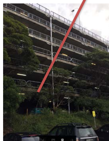
Multi Storey Carpark
