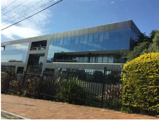
Figure 2.5: 12 Frederick Street (subject site)
