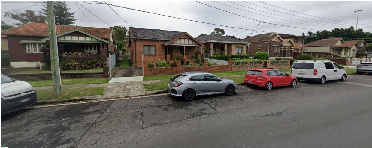
Figure 4 – Character of dwelling houses to be demolished (Gipps Street)
