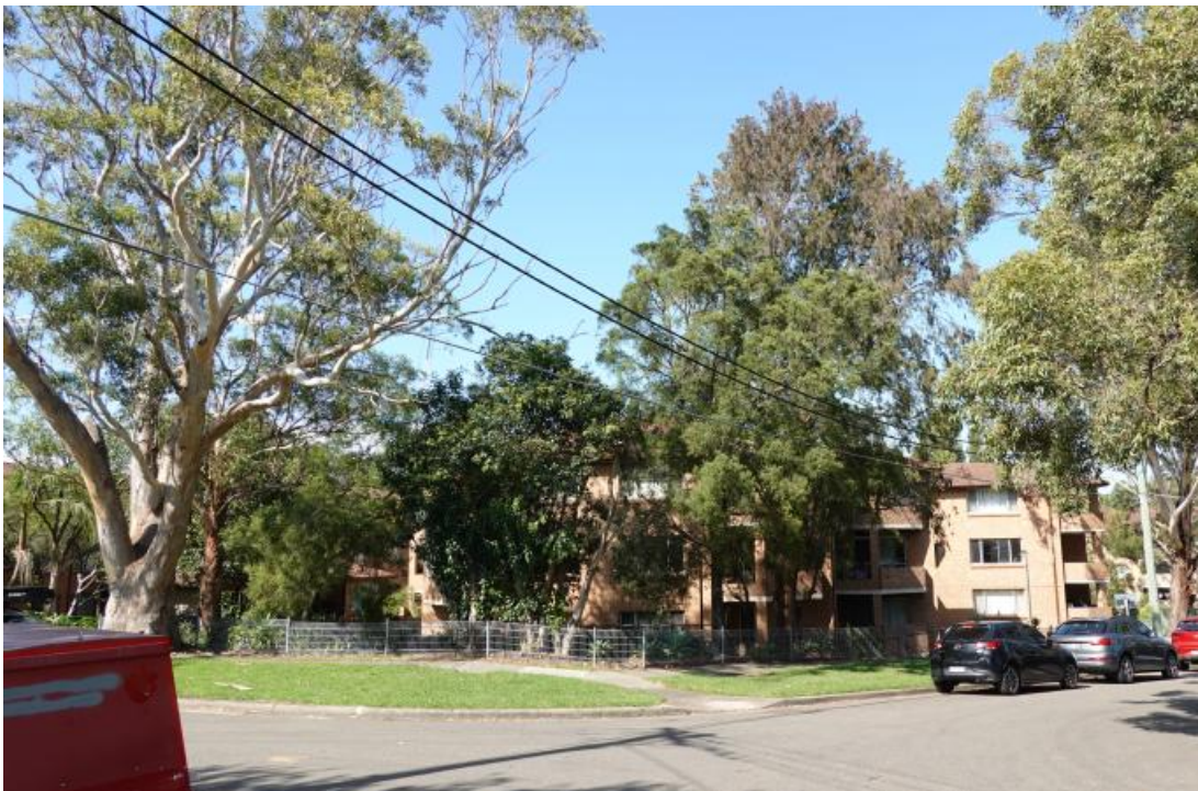
Figure 1.2 – View of the site from the corner of Gardere Street and Flide Street showing the three-storey brick walk-up residential flat buildings with trees of varying retention value fronting the street. (Photo: Arterra 20 March 2025)
