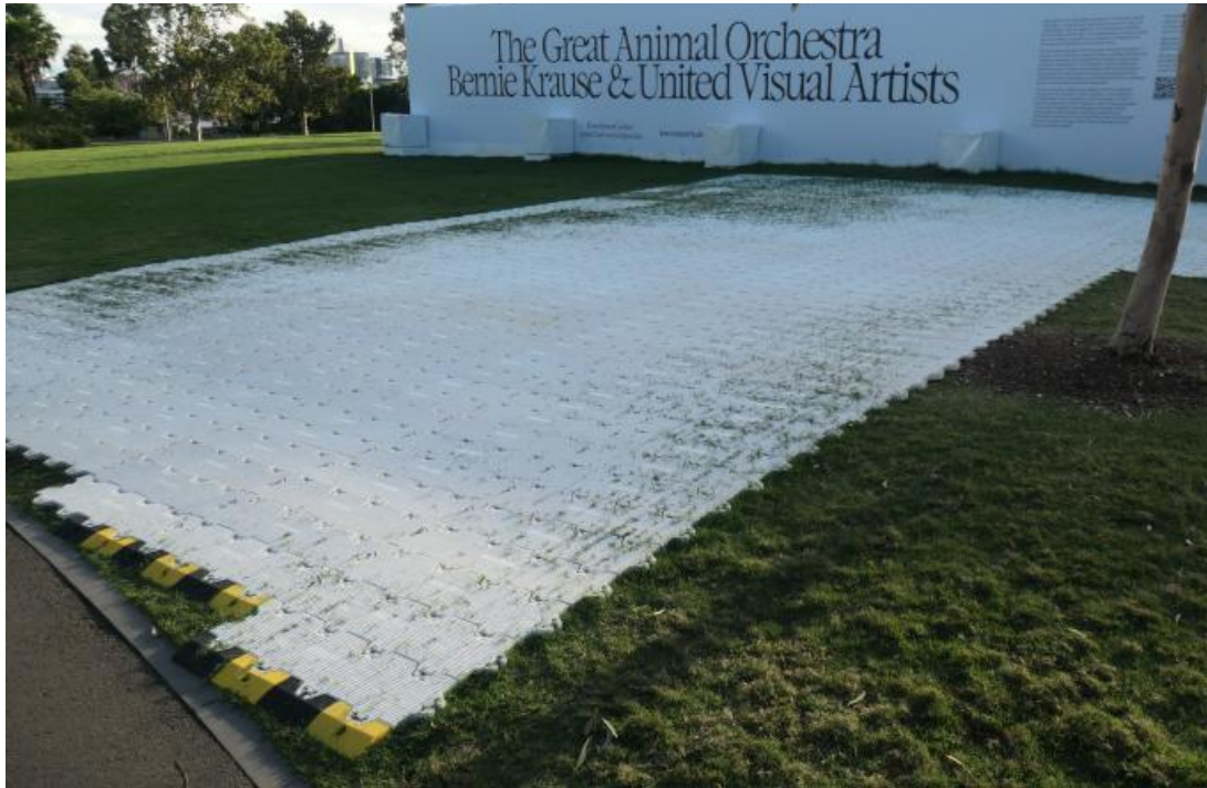
Figure 3.2 – Example of acceptable Tree Protection Area ground protection (Photo: Arterra)
