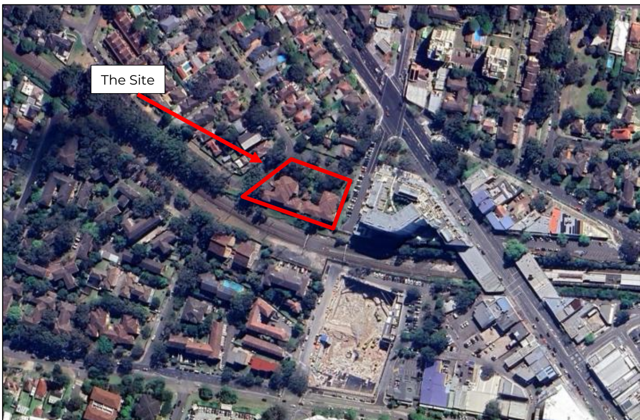
Figure 1: Aerial image of the site location
