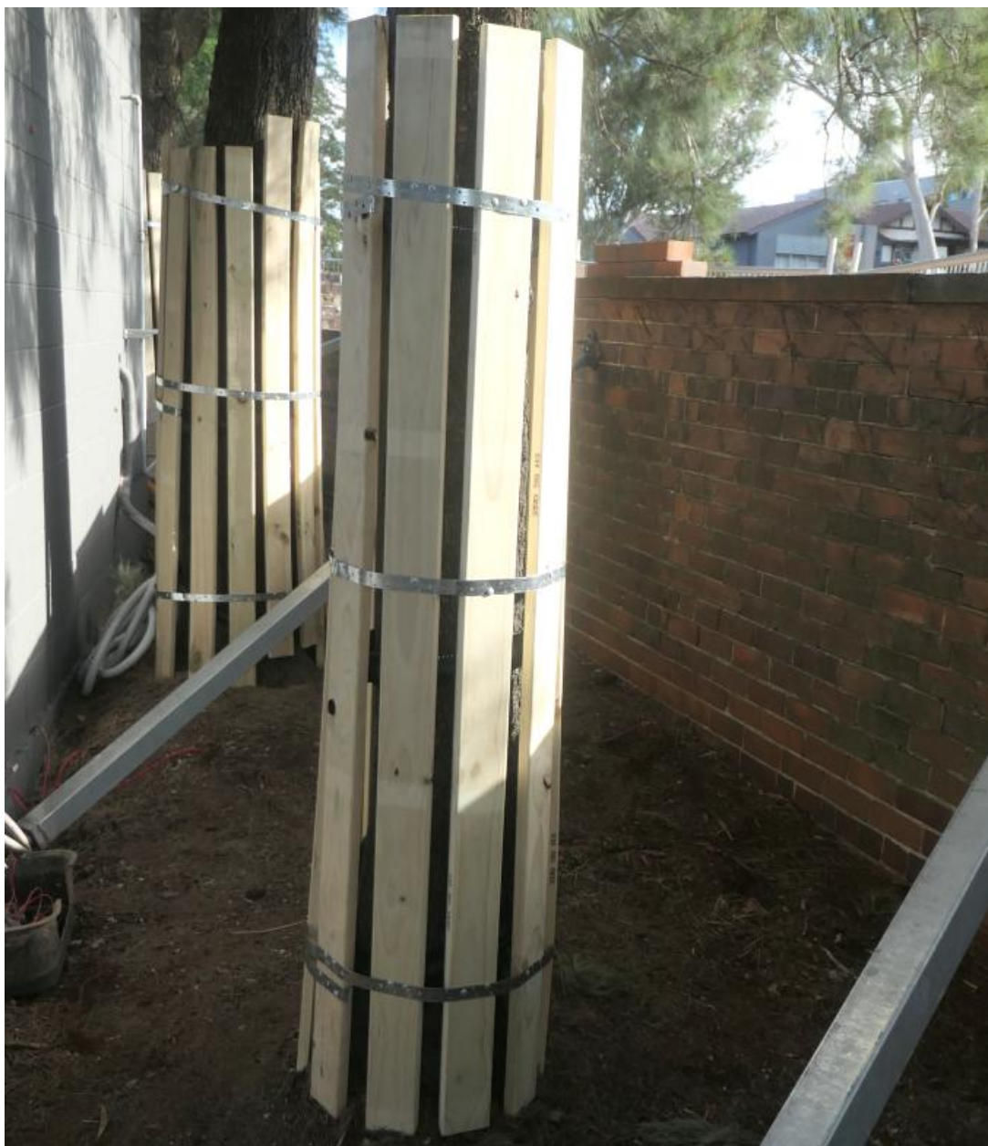
Figure 3.3 – Example of acceptable Trunk Protection batten installation. (Photo: Arterra)
