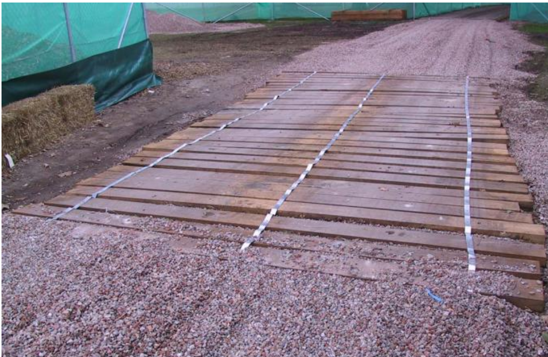
Figure 3.1 – Example of acceptable Tree Protection Area ground protection (Photo: Arterra)
