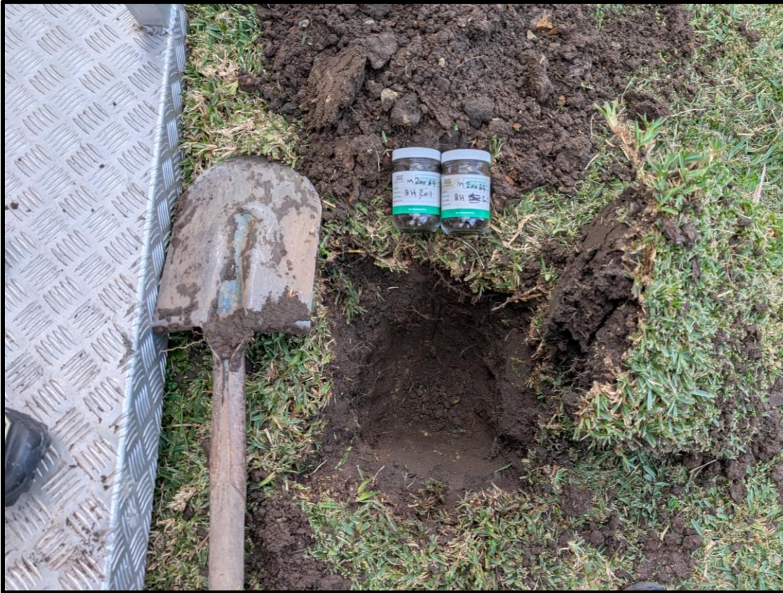
Figure 18. Test pit excavation and sampling of BH20.
