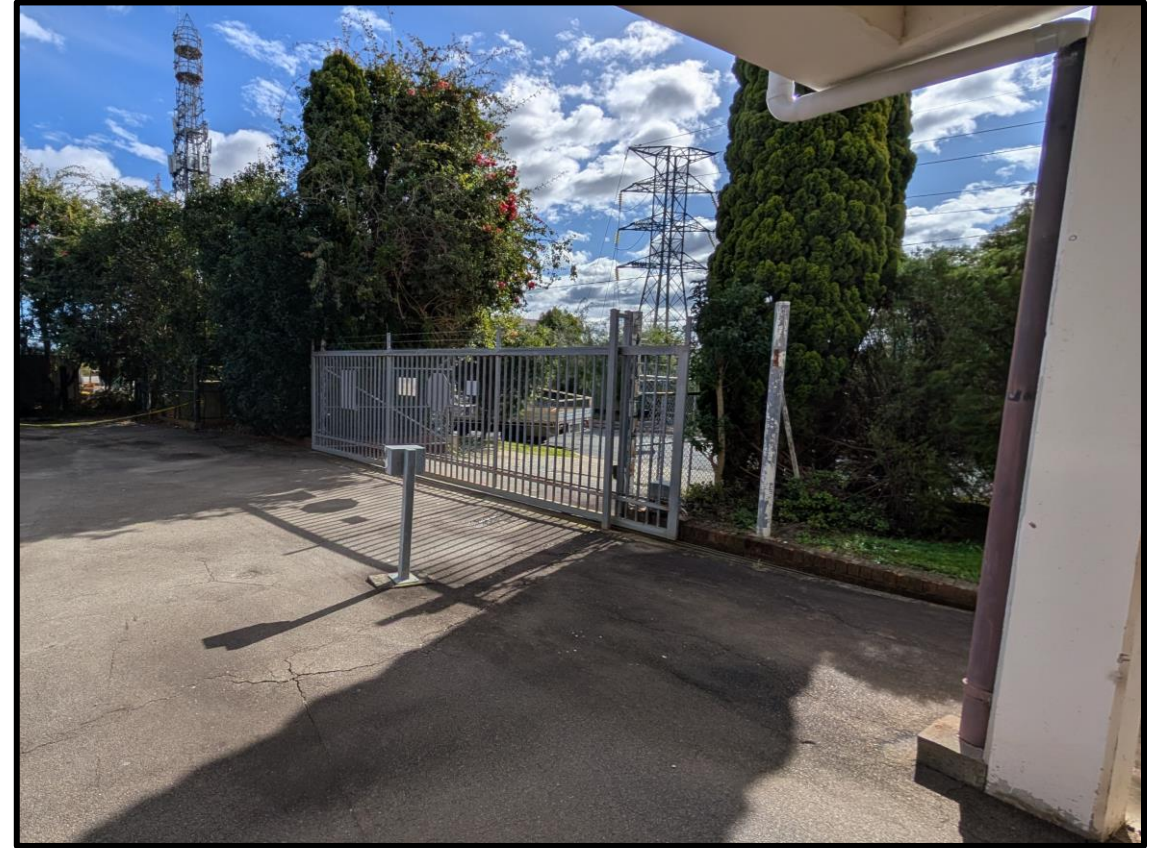
Figure 13. Entrance gate within northwestern portion of the site
