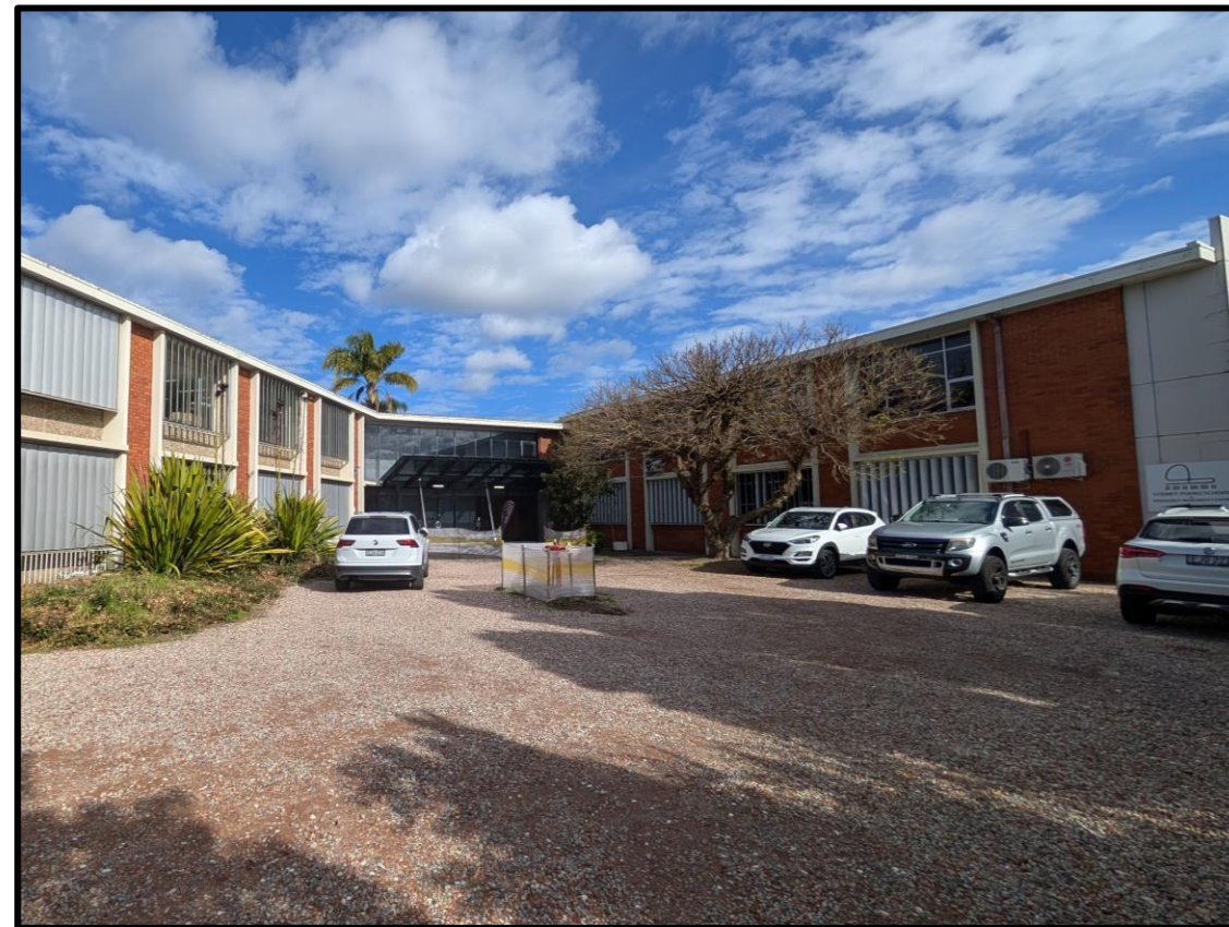
Figure 11. Parking area within northern portion of the site.
