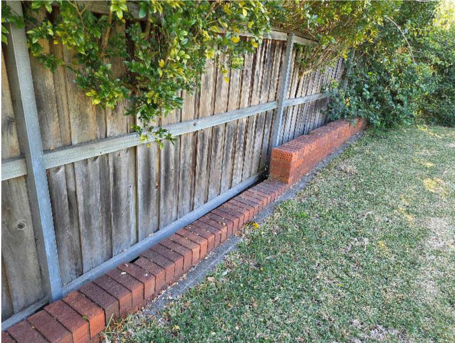
Fig. 80. Photo of retaining wall along Western boundary adjacent T61.
