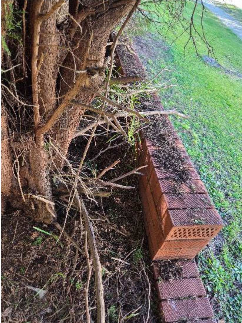
Fig. 14. Photo of T9 adjacent to the front retaining wall.
