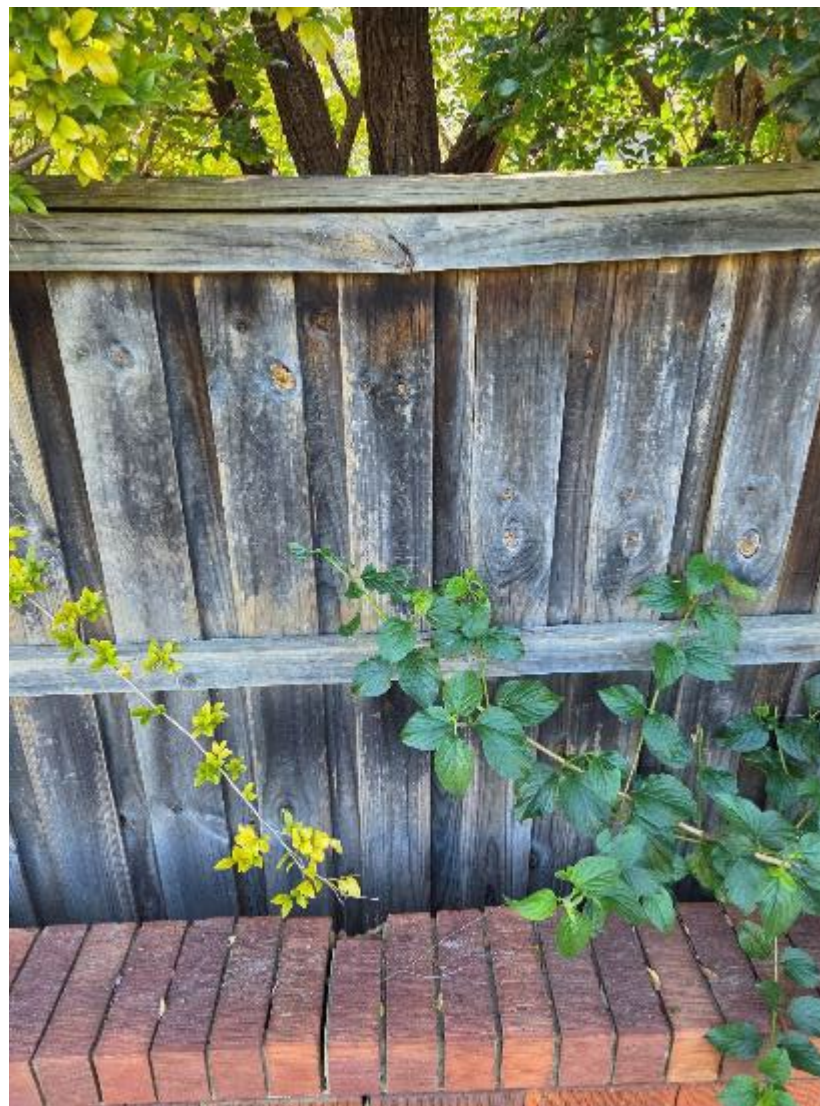
Fig. 84. Photo showing a brick retaining wall on the Western border of the Site.
