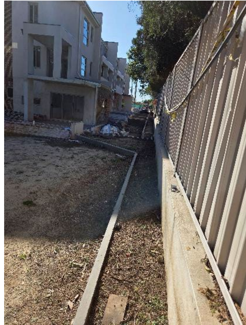
Fig. 73. Photo of a timber retaining wall and fence adjacent to trees T56, T57 & T58.
