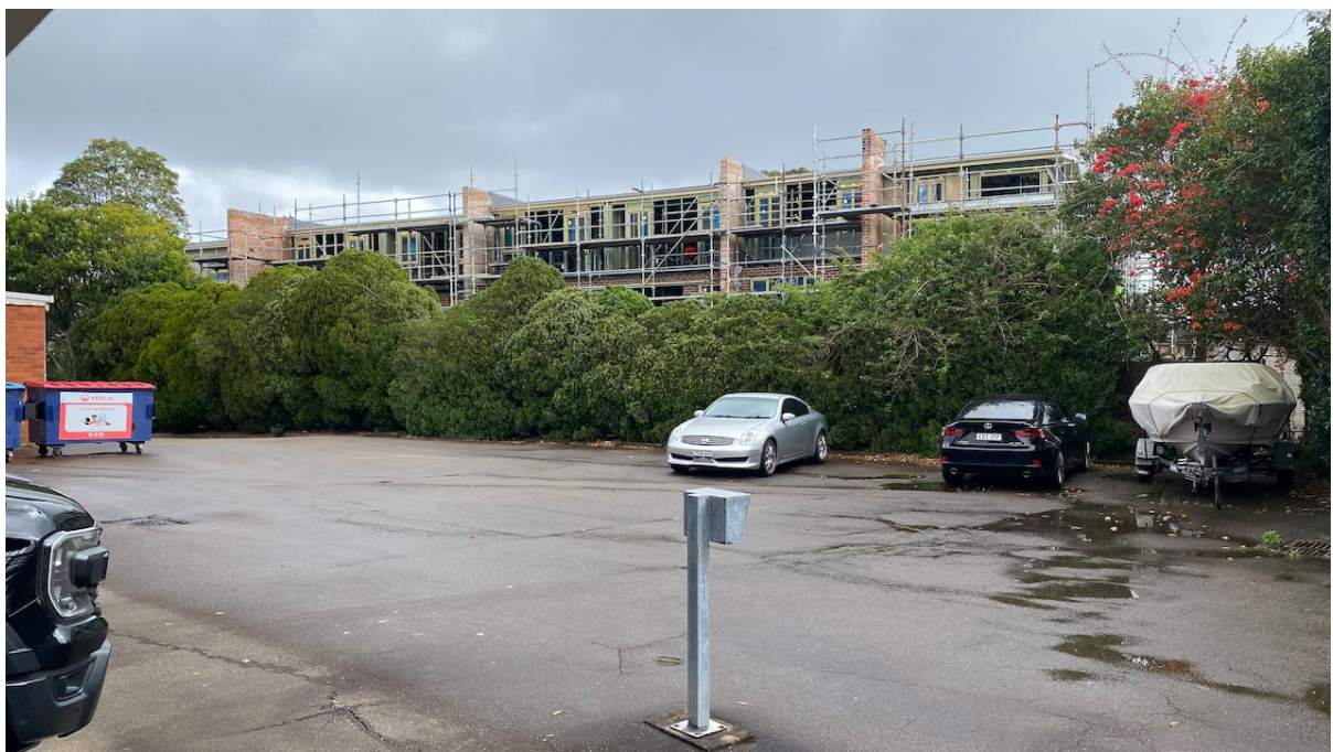
Plate 20. Construction of new residential buildings along the west of the site. (Source: Heritage Now 2024)
