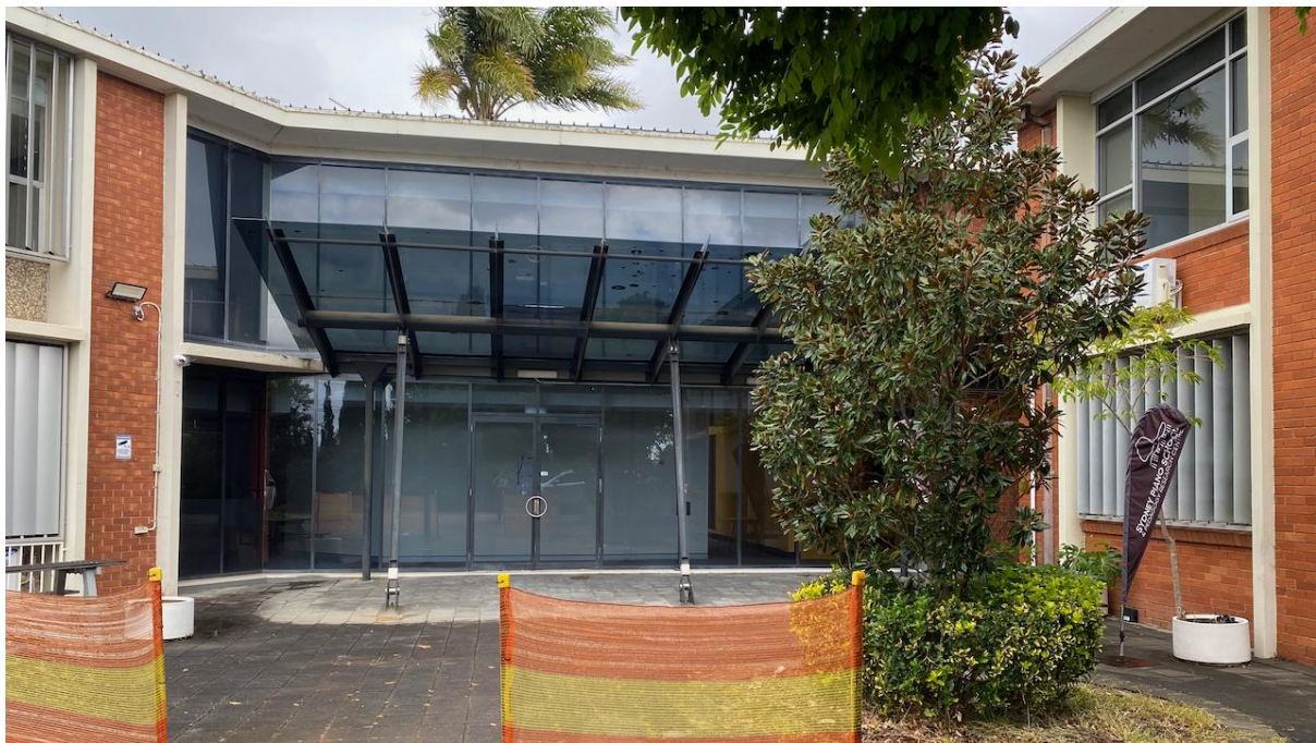
Plate 18. Rear of building facing Felton Street, showing a glass entrance and paved area. (Source: Heritage Now 2024)
