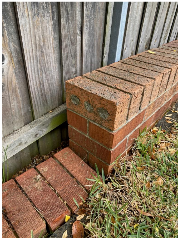
Plate 4. Machine-made brick retaining wall present around whole of property. (Source: Heritage Now 2024)
