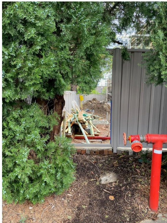
Plate 14. Gap through fencing showing the drop down to the west in the adjacent property. (Source: Heritage Now 2024)
