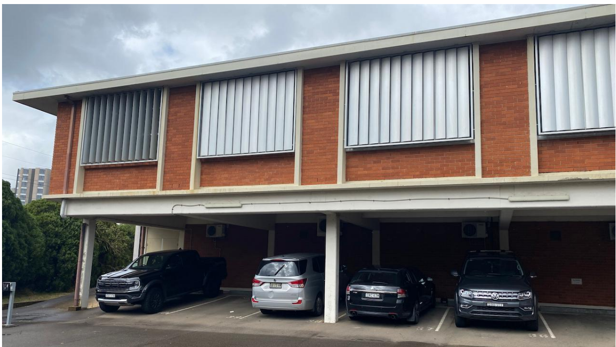
Plate 16. North-western corner of site used as a carpark. Brick building with large, shuttered windows present. (Source: Heritage Now 2024)
