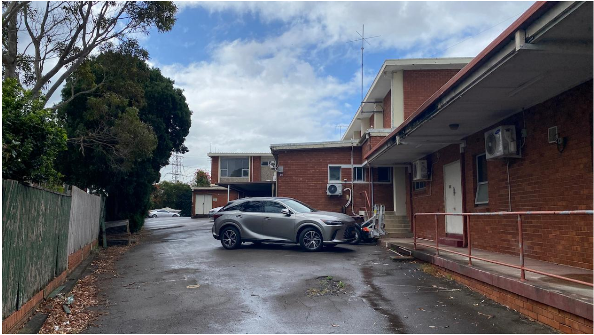
Plate 9. Western side of building, showing the use of the orange machine-made bricks. (Source: Heritage Now 2024)
