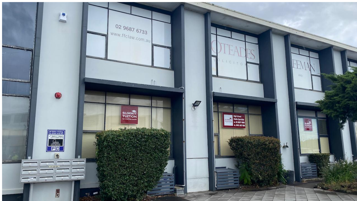
Plate 7. Windows and signage of building facing onto Pennant Hills Road. (Source: Heritage Now 2024)
