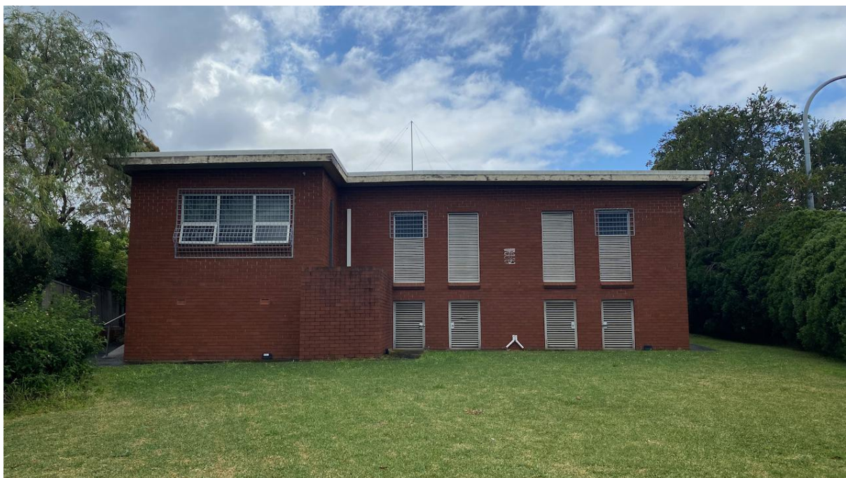
Plate 8. South-western part of the building that was constructed using exposed orange machine-made bricks. (Source: Heritage Now 2024)
