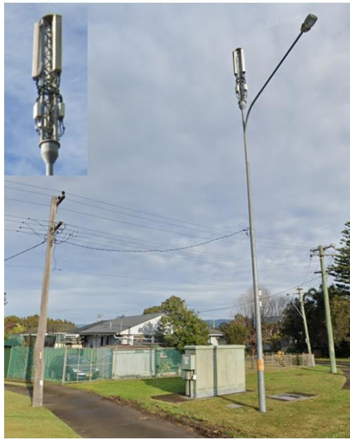
Telecommunications equipment on the road verge and streetlight column in Bedford Street and Northcliffe Drive, Berkeley. Source: Google Maps Street View.
