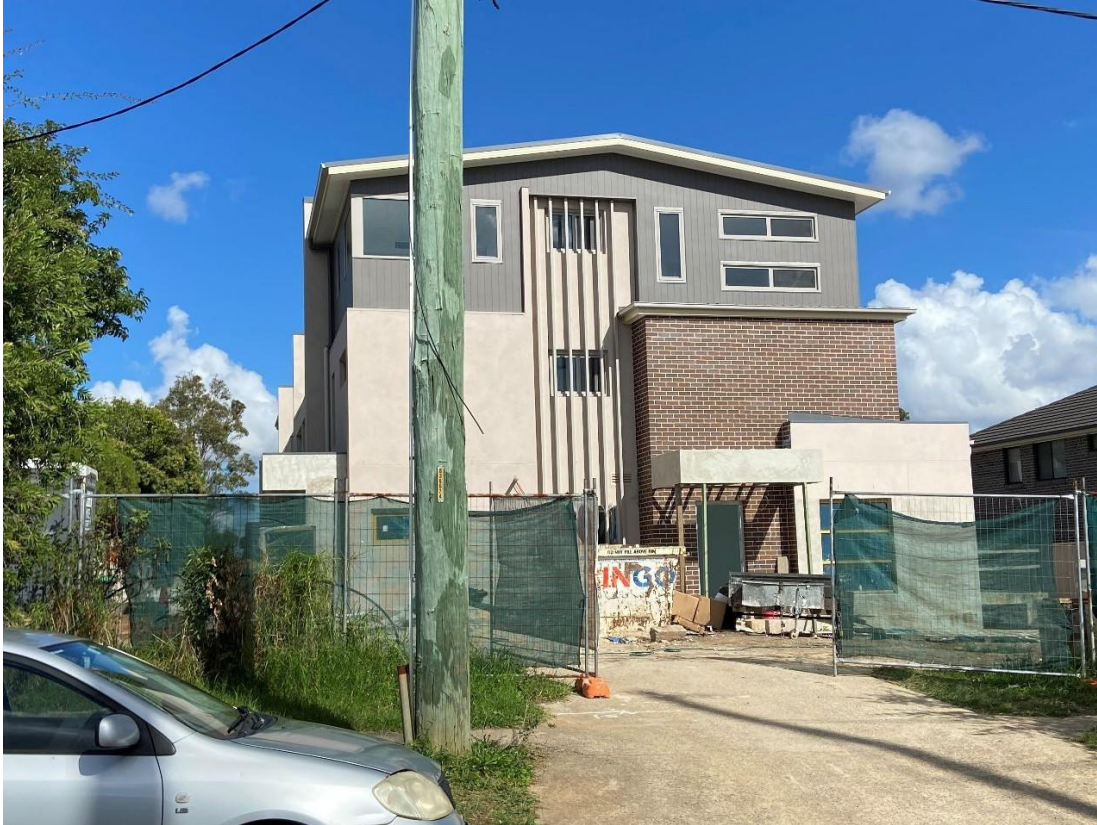
View of the adjoining residential building adjoining the site in Felton Road
