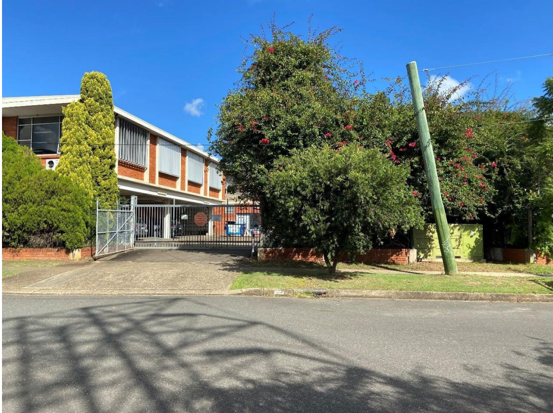
View from Felton Road of the existing driveway access and substation
