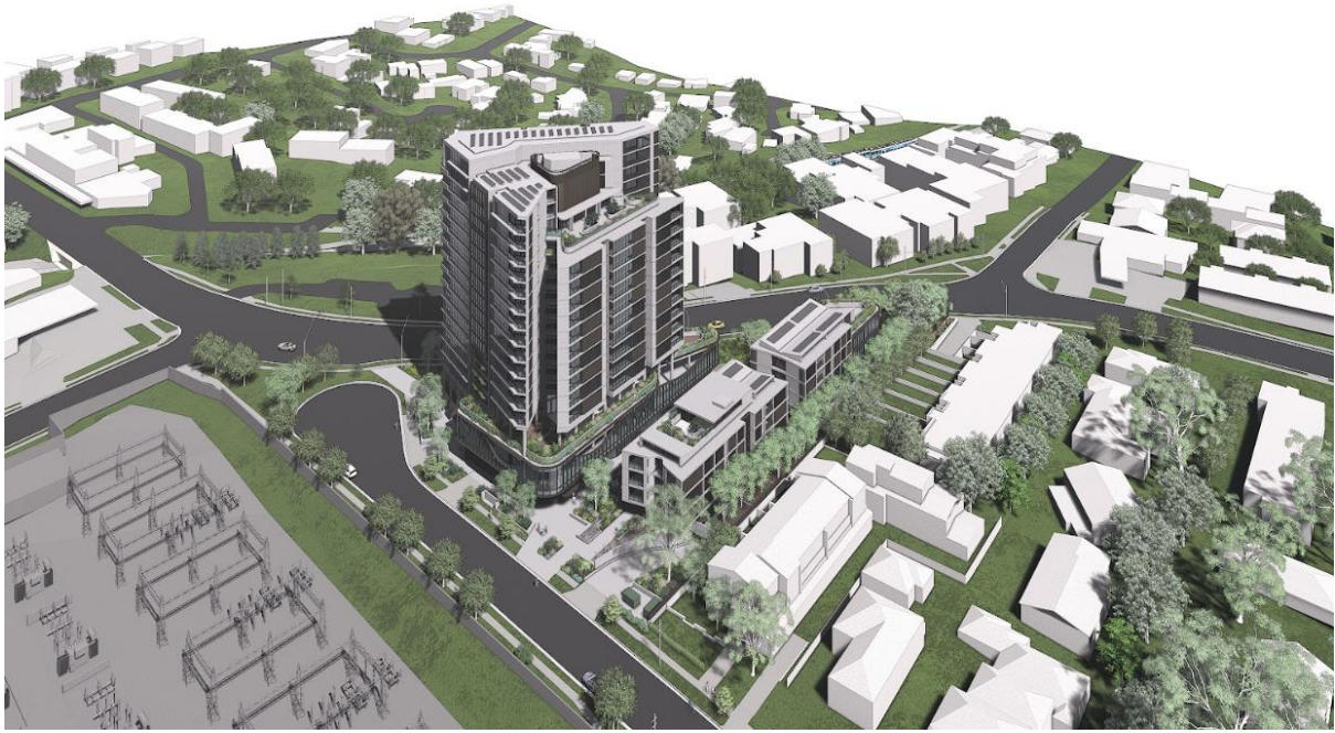
View of the development in its local context
