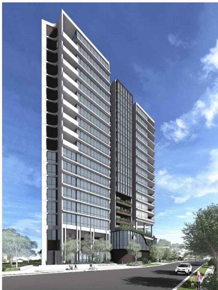
View of the development as viewed from the head of the cul de sac in Felton Road
