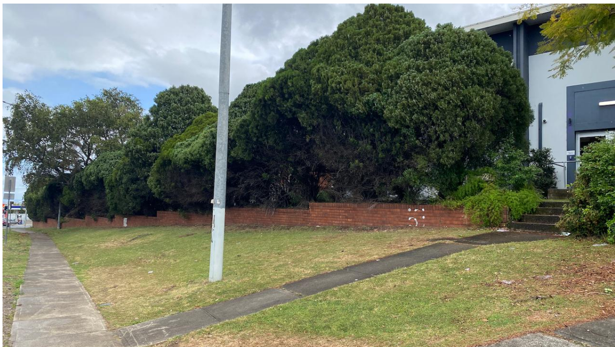
Plate 7. Part of the retaining wall that surrounds the Project Area. (Source: Heritage Now 2024)
