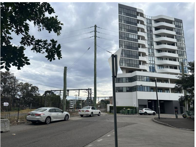
Figure 12. Shop top housing to the southwest of site (1 Treacy Street) (Source: PPUD, 2025)
