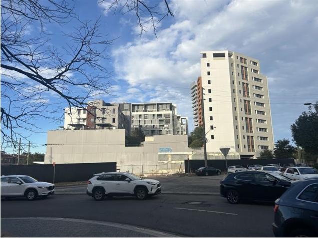
Figure 8. Frontage of subject site (Hill Street) (Source: PPUD, 2025)
