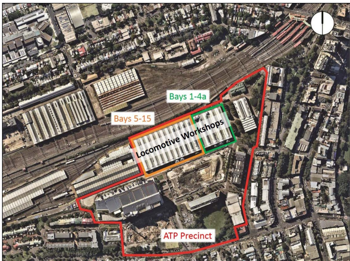
Figure 2 | Aerial view of Locomotive Workshop and ATP
