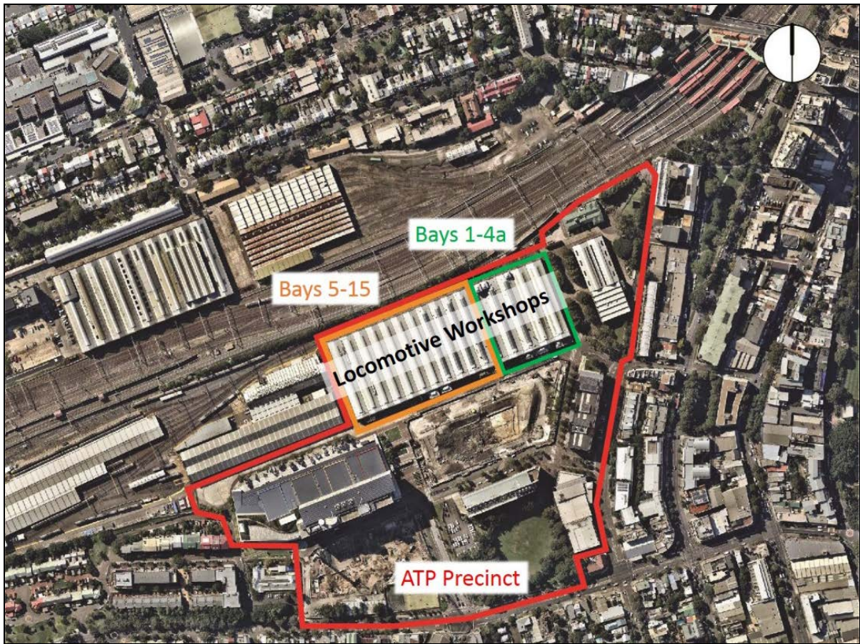
Figure 2 | Aerial view of Locomotive Workshop and ATP
