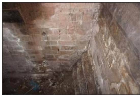
Figure 7 | Photo of Bay 15 brick pit after partial removal of modern steel plates (Source: Curio Projects)
