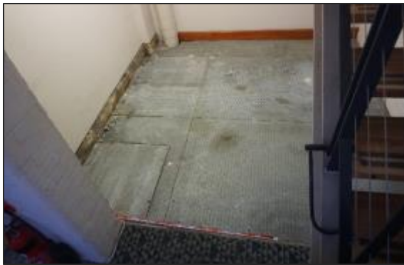
Figure 6 | Photo of Bay 15 brick pit with modern steel plates covering the brick pit (Source: Curio Projects)
