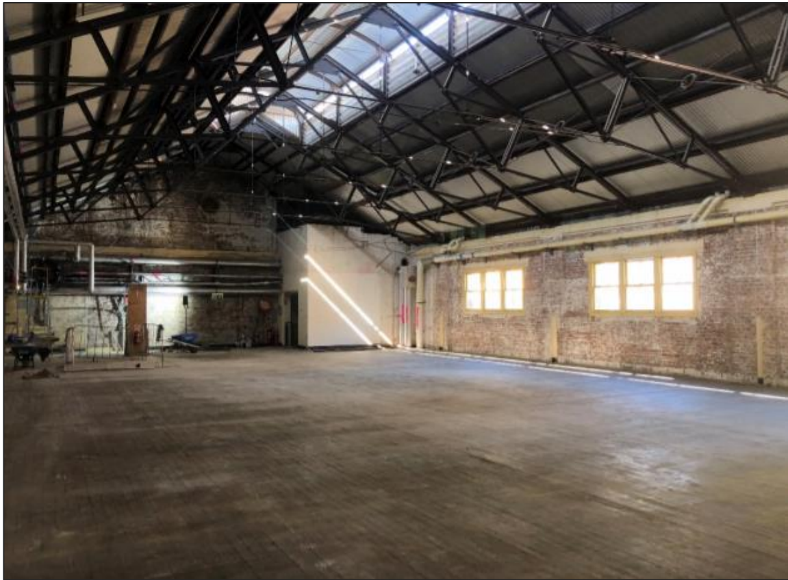
Figure 5 | Photo of Bay 15 South mezzanine platform (Source: Curio Projects)
