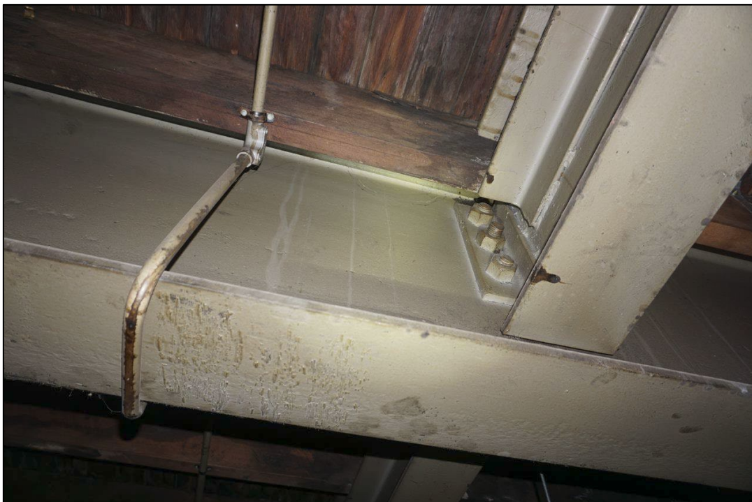
Figure 5.2: Steel beams running east to west are screwed and bolted onto steel columns running north to south. Mezzanine floorboards also in view. Source: Curio Projects, 2020
