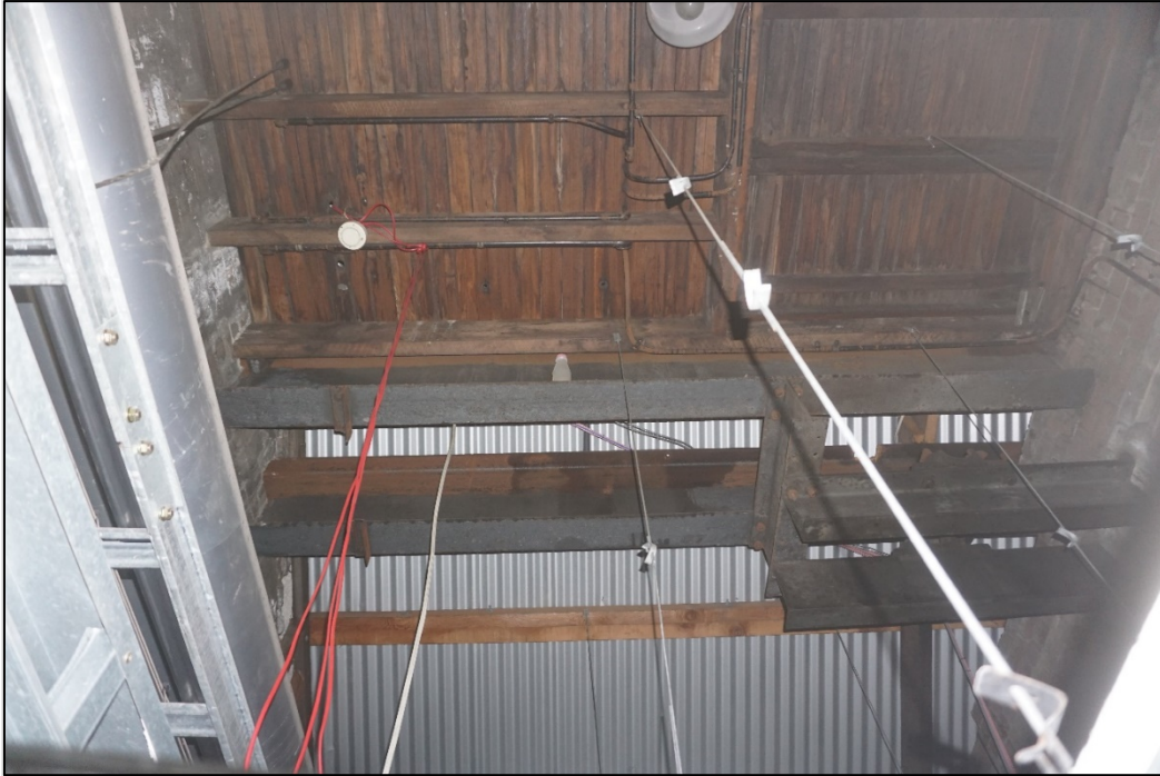
Figure 5.19: Steel and timber structure associated with potential hoist mechanism on top of the east to west brick wall at the southwest corner of Bay 15.
