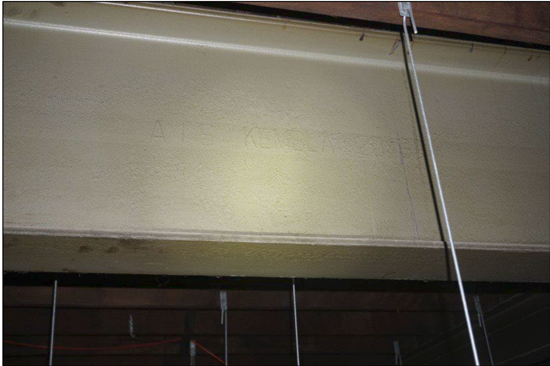
Figure 5.7: Close up of steel beam with 'A.I.S KEMBLA 20X**' inscription. Source: Curio Projects, 2020
