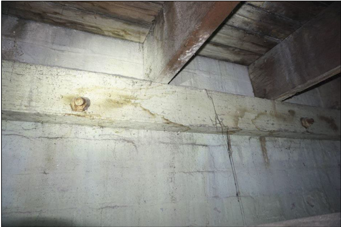
Figure 5.5: A closeup of narrower and intersecting timber floorboards acting as bearers, then timber joists, which are the base of the mezzanine platform floorboards (east wall). Source: Curio Projects, 2020
