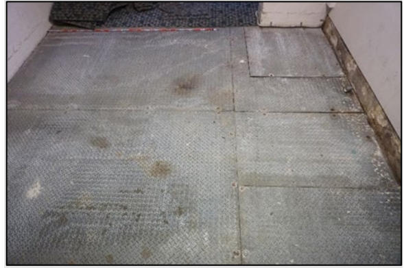
Figure 5.16: Current modern steel plates covering brick pit in southwest corner of Bay 15. Source: Curio Projects, 2020
