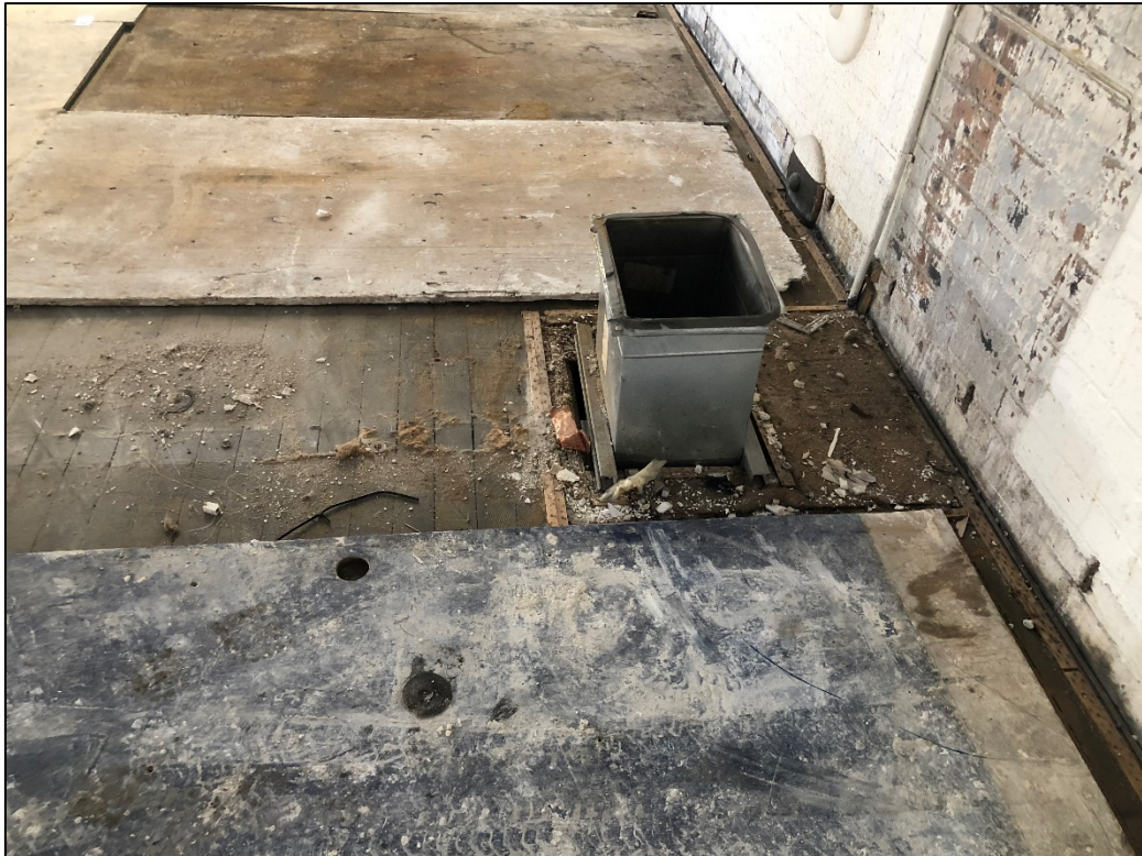
Figure 5.12: Existing penetration on mezzanine platform. Source: Curio Projects, 2020
