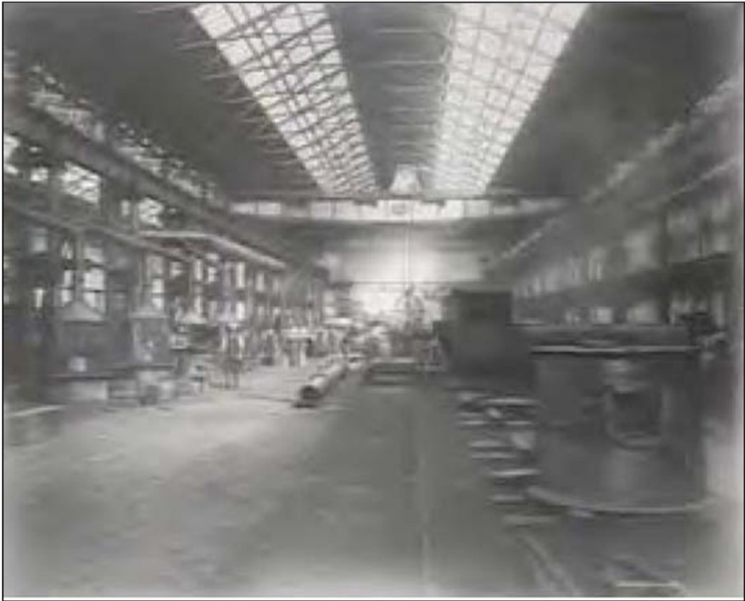
Figure 3.1: Interior of the Locomotive Workshops, date Unknown. (Source: Government Printing Office Collection, State Library of NSW)
