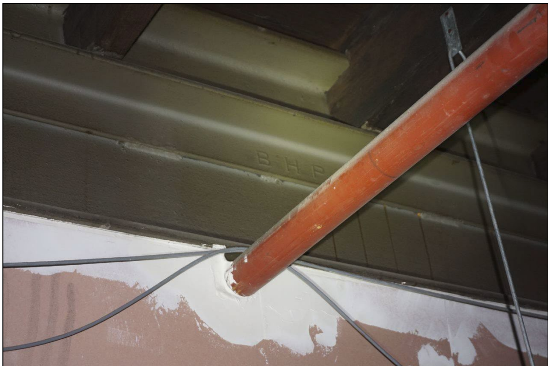
Figure 5.6: Closeup of steel beam with 'BHP' inscription. Source: Curio Projects, 2020
