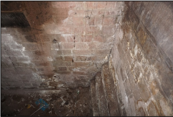
Figure 5.17: Brick pit after partial removal of modern steel plates in southwest corner of Bay 15. Source: Curio Projects 2020
