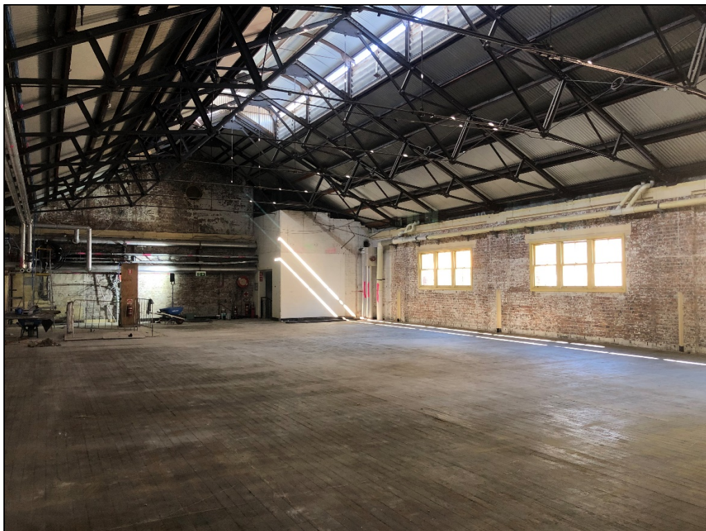
Figure 5.9: Bay 15 South mezzanine platform. Western brick wall to the right; potential hoist/lift structure and brick wall at the back. Source: Curio Projects, 2020
