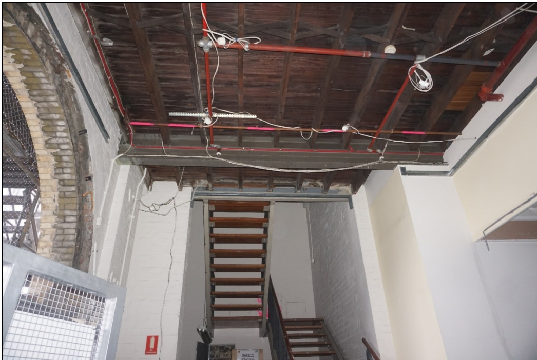
Figure 5.20: East to west brick wall and adjoining timber platform at the southwest corner of Bay 15. Modern staircase occupies the space potentially used as a hoist/lift.
