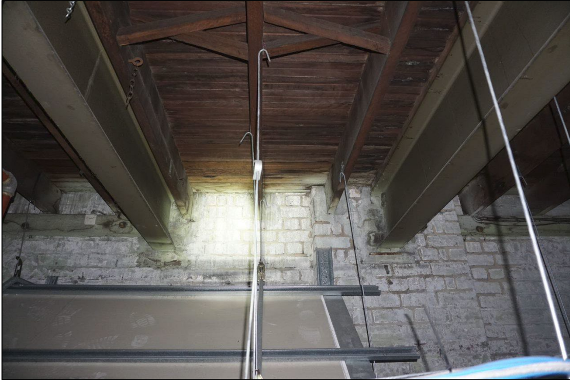
Figure 5.3: Steel beams aligned east-west abutting Bay 15 South western brick wall. Narrower 'crisscrossing' timber floorboards between the north-south floorboards of the mezzanine platform. Source: Curio Projects, 2020
