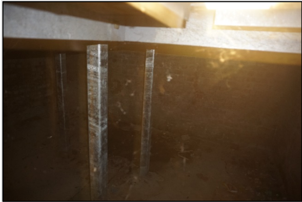
Figure 5.18: Brick pit after partial removal of modern steel plates in southwest corner of Bay 15. Source: Curio Projects 2020
