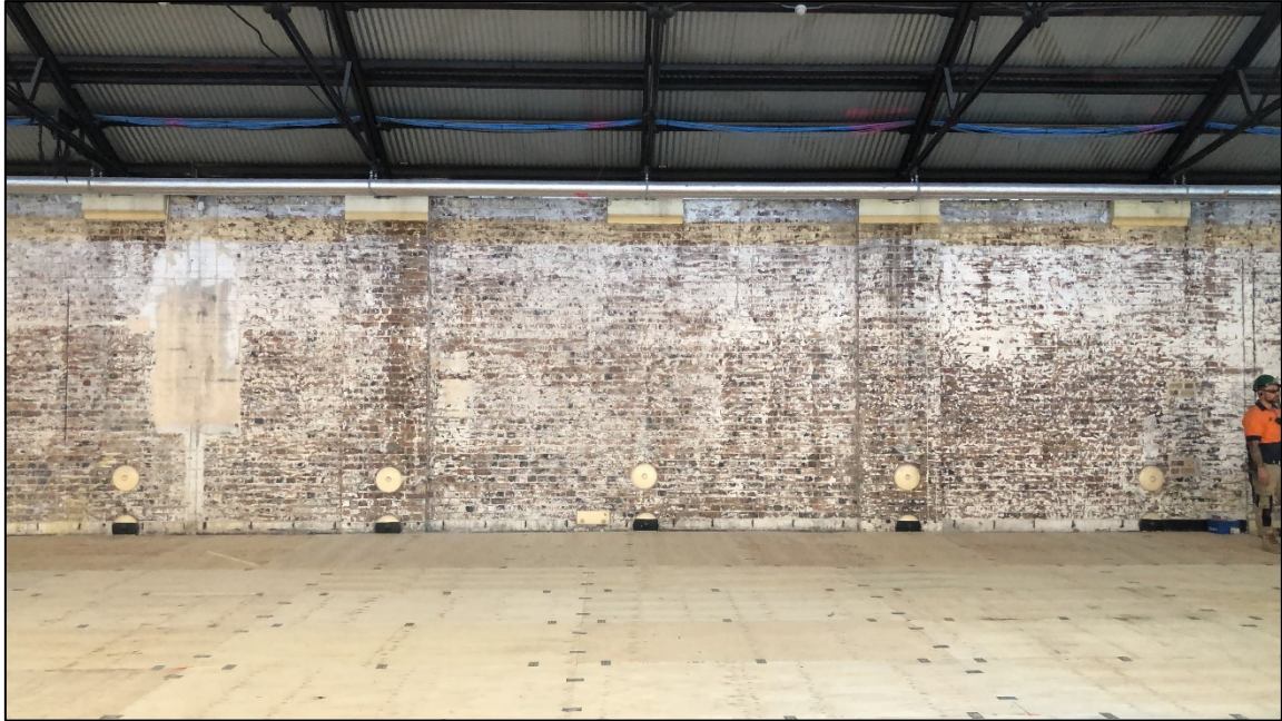
Figure 5.10: Eastern brick wall and sandstone details. Source: Curio Projects, 2020
