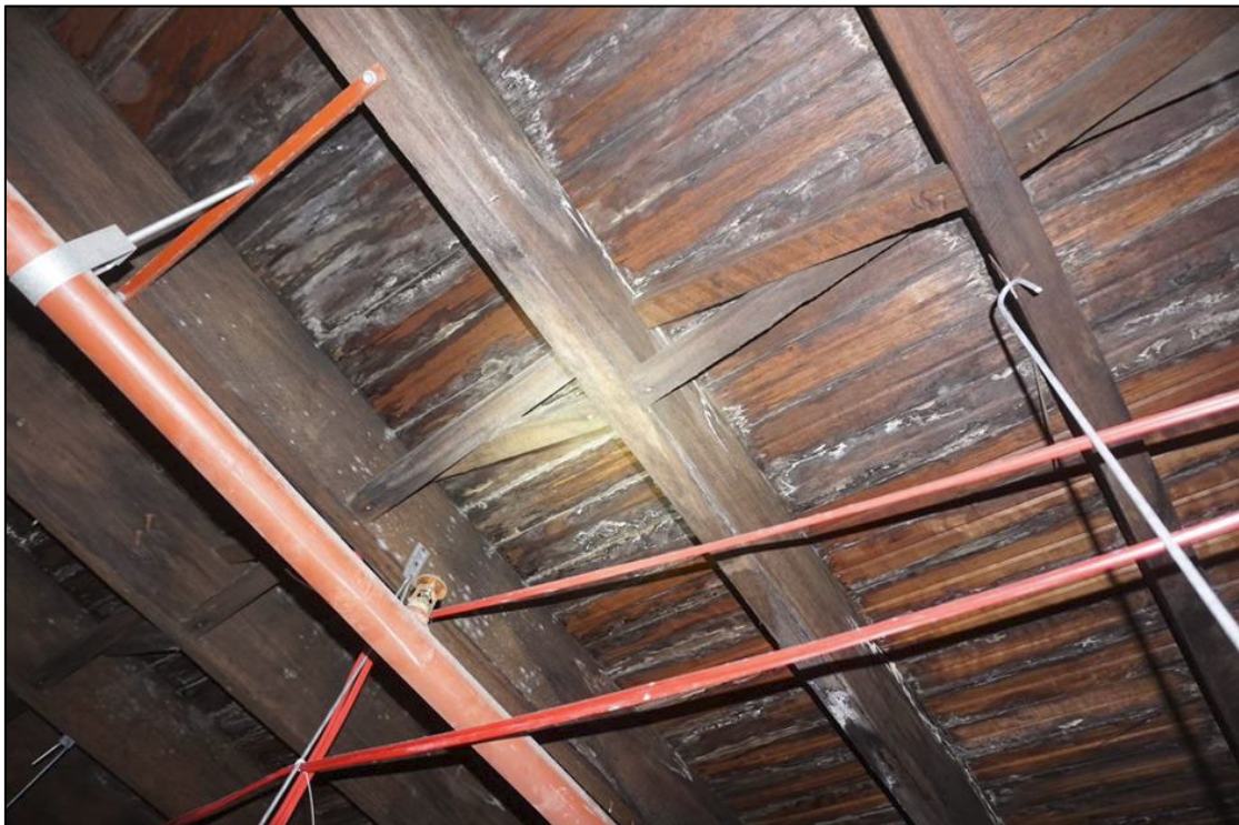
Figure 5.4: Narrower timber-cross brace between the north-south floorboards of the mezzanine platform. Source: Curio Projects, 2020
