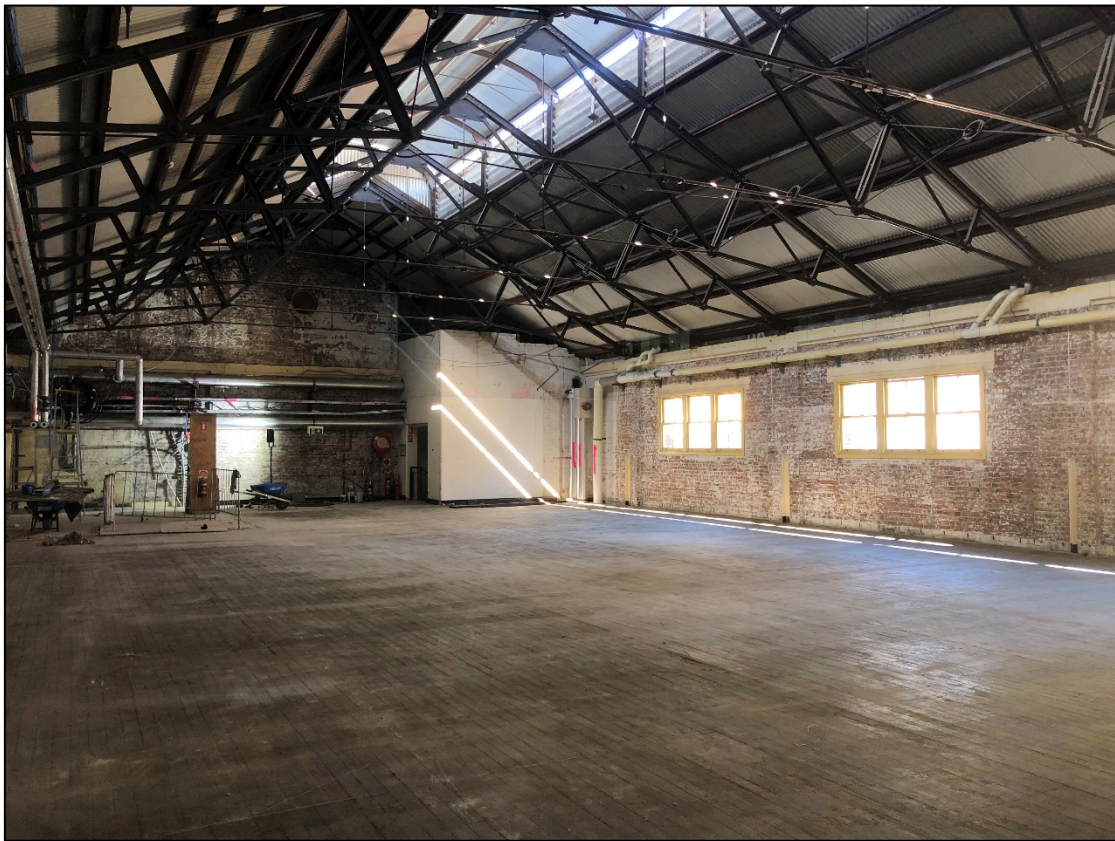
Figure 5.14: Brick wall at the southwest corner associated with a potential hoist/lift mechanism. Source: Curio Projects, 2020
