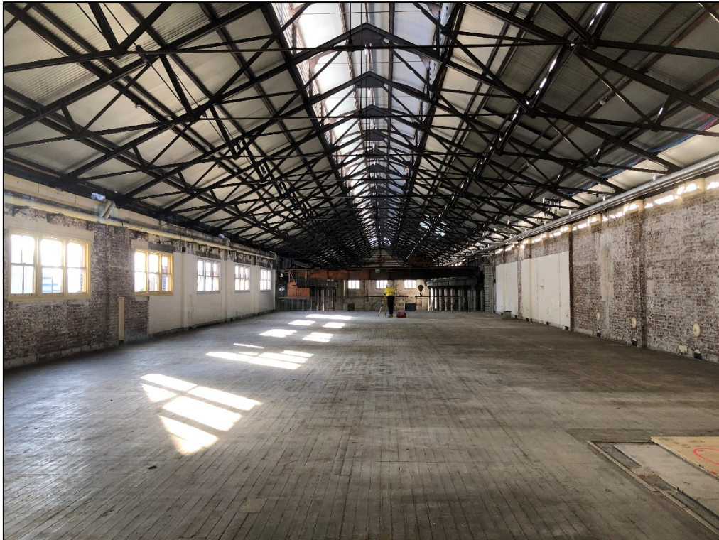
Figure 5.8: Bay 15 South mezzanine platform. Source: Curio Projects, 2020
