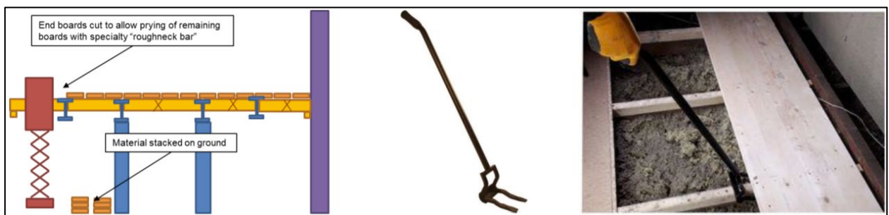
Figure 6.2: Dismantling process of the timber floorboards Source: Mirvac, 2020
