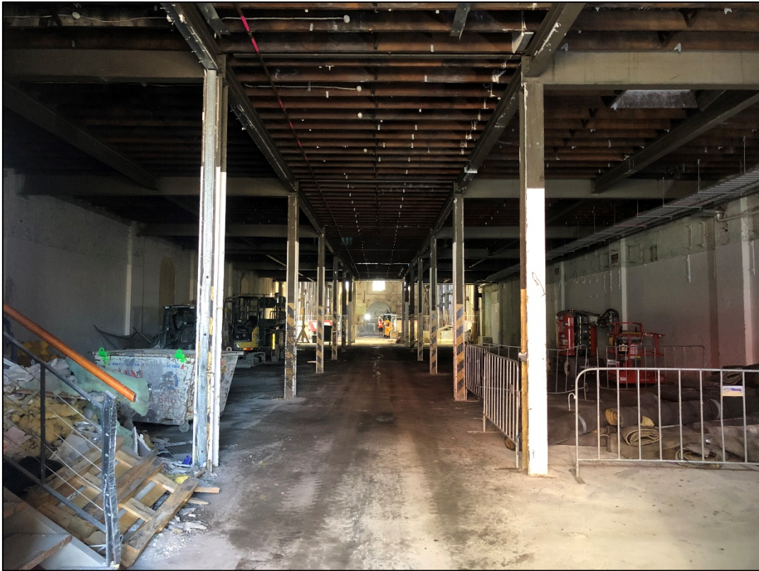
Figure 5.1: Ground Floor of Bay 15 South after the removal of the 1990s fit-out. Source: Curio Projects, 2020
