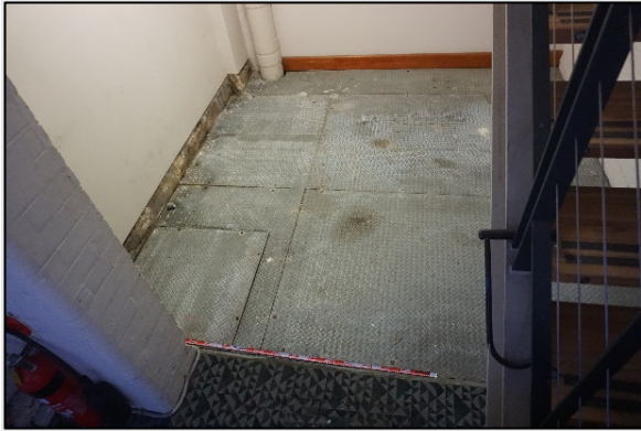
Figure 5.15: Modern steel plates covering brick pit in southwest corner of Bay 15. Source: Curio Projects, 2020
