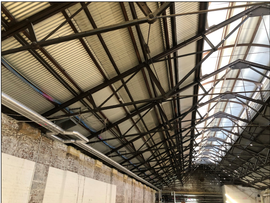
Figure 5.11: Bay 15 original steel roof, eastern brick wall and sandstone details. Source: Curio Projects, 2020
