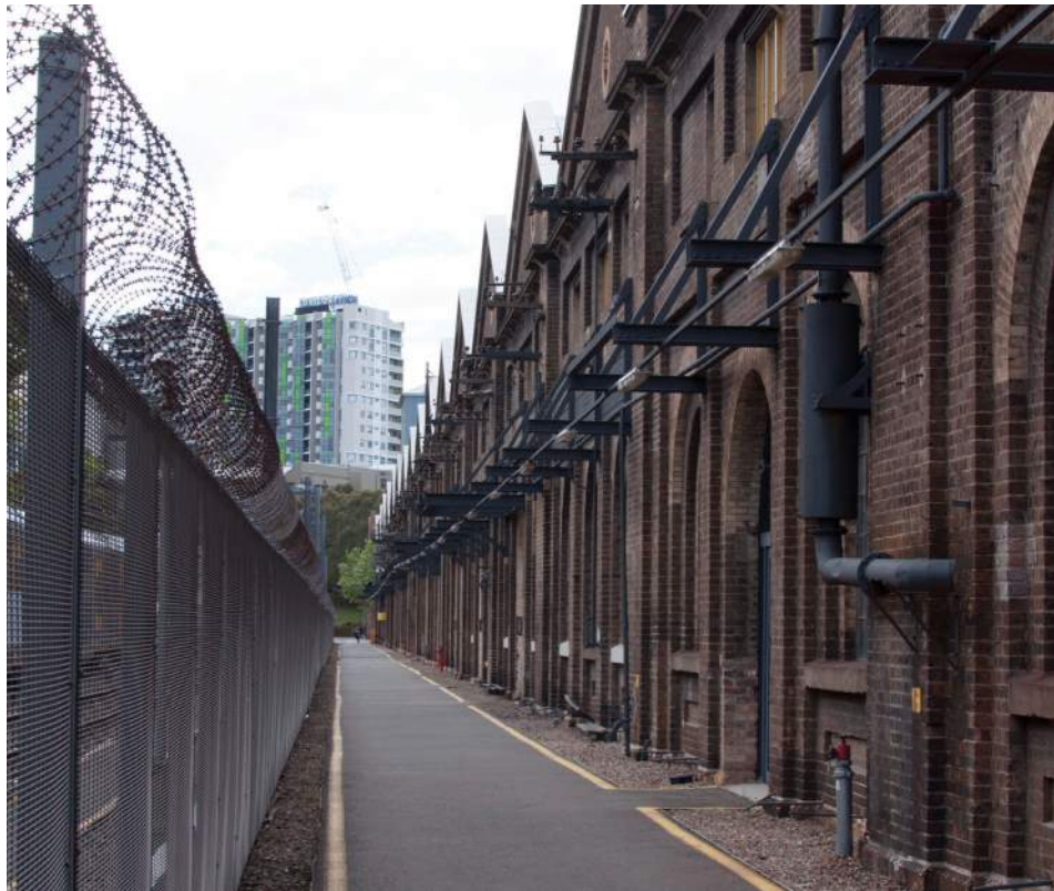
Northern Right of Way, looking east
