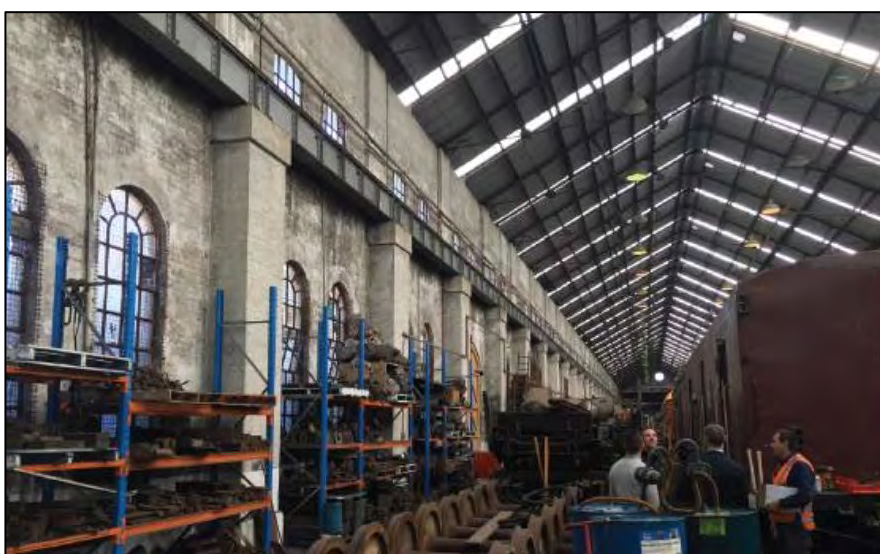
FIGURE 54: ROOF PROFILE OF THE LARGE ERECTING SHED (SOURCE: ETHOS URBAN)
