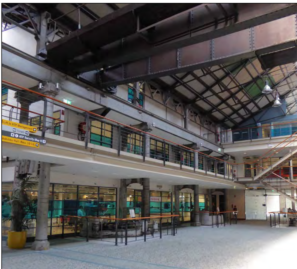
FIGURE 68: AN EXAMPLE OF THE 1990S THREE-STOREY MODERN INFILL PROPOSED TO BE DEMOLISHED IN BAY 5 (SOURCE: CURIO 2017)
