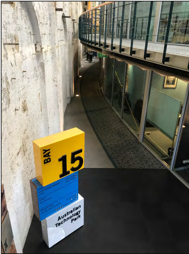
FIGURE 23: EXTANT WALL BETWEEN BAYS 14 AND 15, FACING WEST, (SOURCE: ETHOS URBAN 2017)
