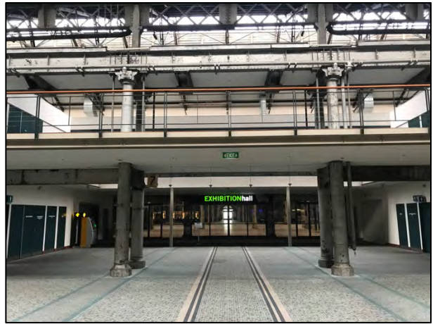
FIGURE 20: MEZZANINE LEVEL ACROSS BAY 8, VIEW WESTERN TO ENTRANCE TO EXHIBITION HALL IN BAYS 9-13 (SOURCE: ETHOS URBAN 2016)
