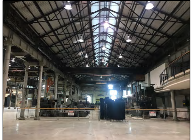
FIGURE 82: MACHINERY IN BAY 9 NORTH, 'ACCESS PATH' FILLED WITH EXHIBITION CENTRE EQUIPMENT (SOURCE: ETHOS URBAN 2017)
