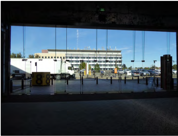
FIGURE 19: GLASS OPENING AT SOUTHERN END OF BAY 7 (SOURCE: CURIO 2016)
