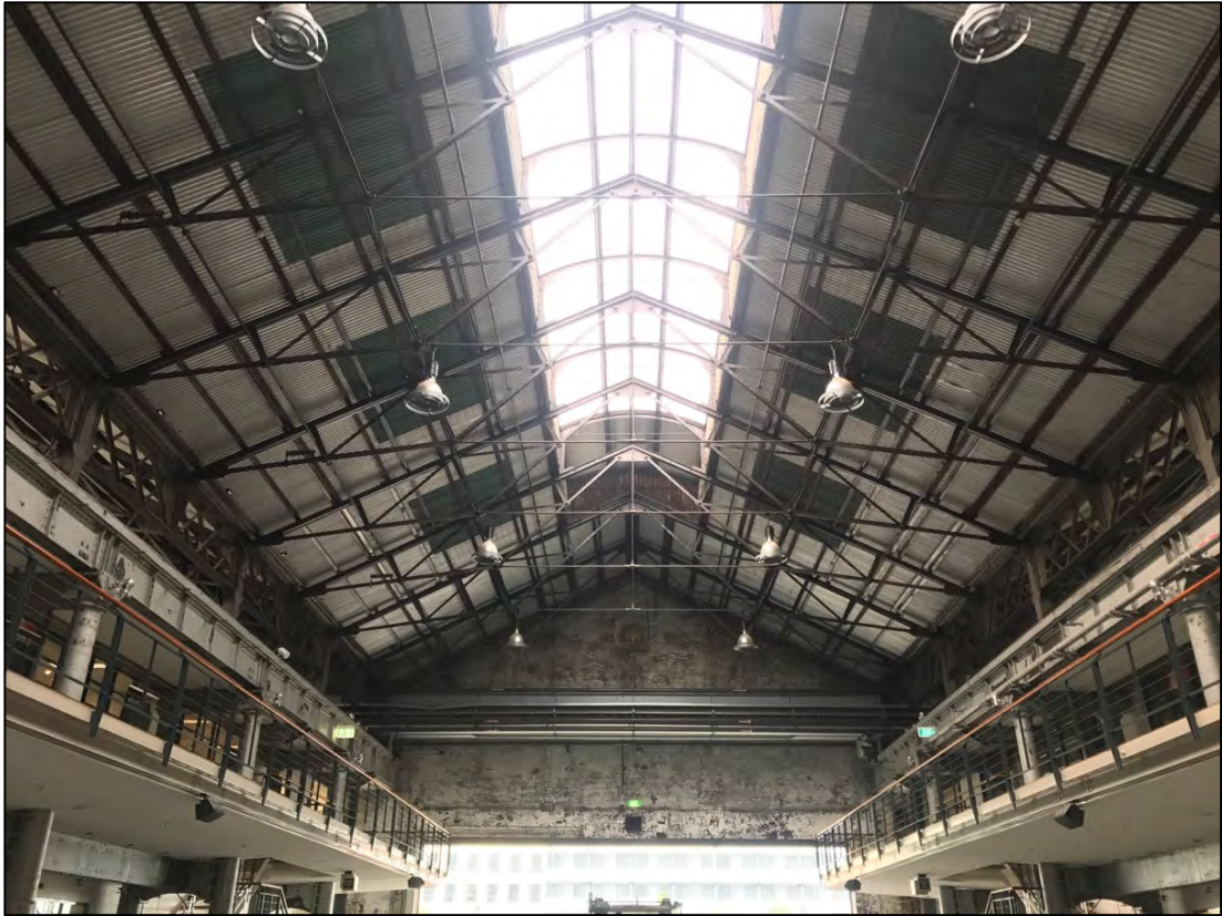
FIGURE 58: EXISTING POLYCARBONATE CURVED LANTERN ROOF FORMAT IN BAY 7 (SOURCE: ETHOS URBAN 2017)
