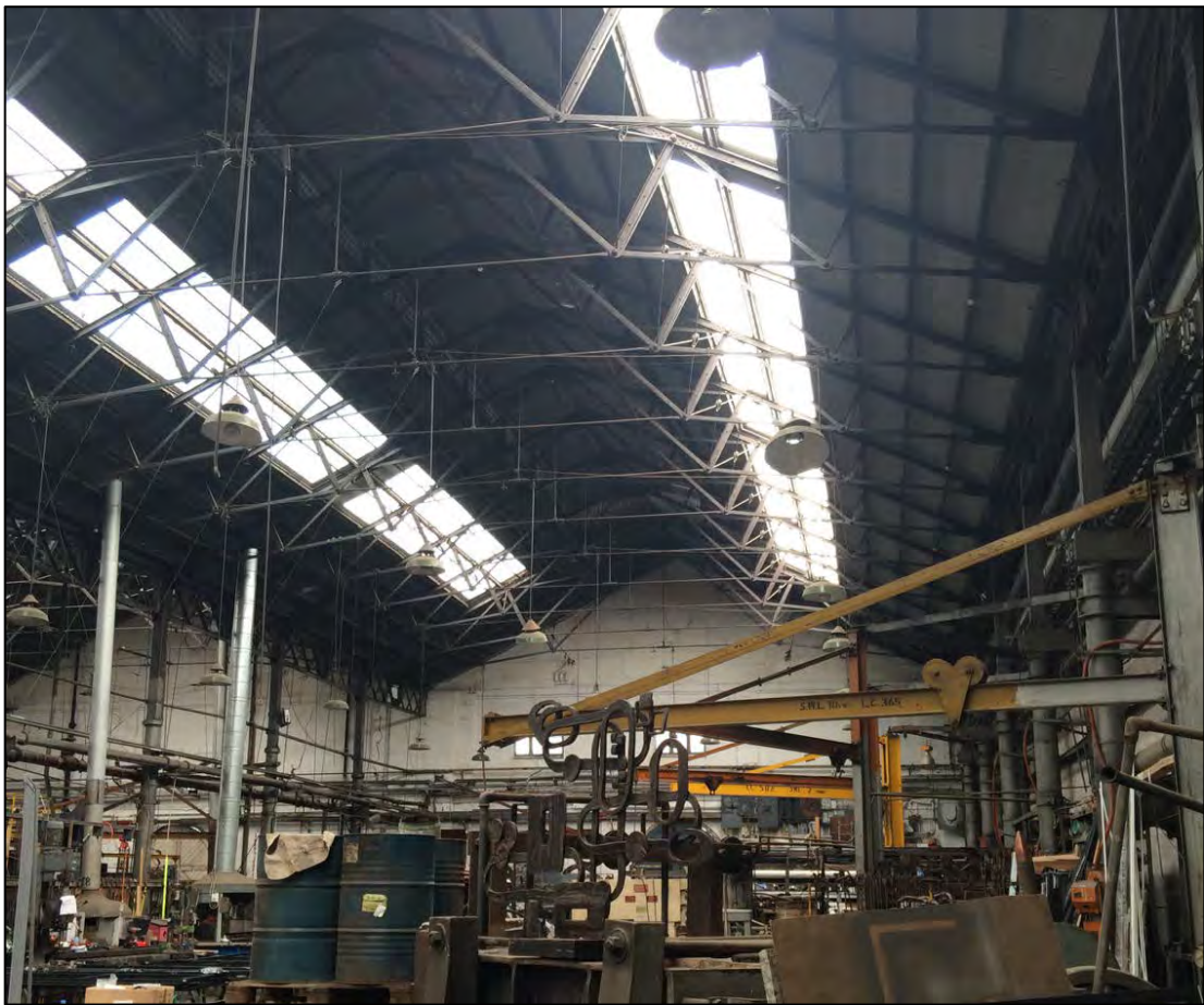
FIGURE 59: EXISTING ROOF IN BAYS 1 AND 2 (SOURCE: CURIO 2016)
