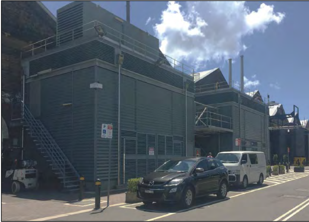
FIGURE 71: EXISTING SUBSTATION TREATMENT AT TWO OF THE SUBSTATIONS (SOURCE: SISSONS)
