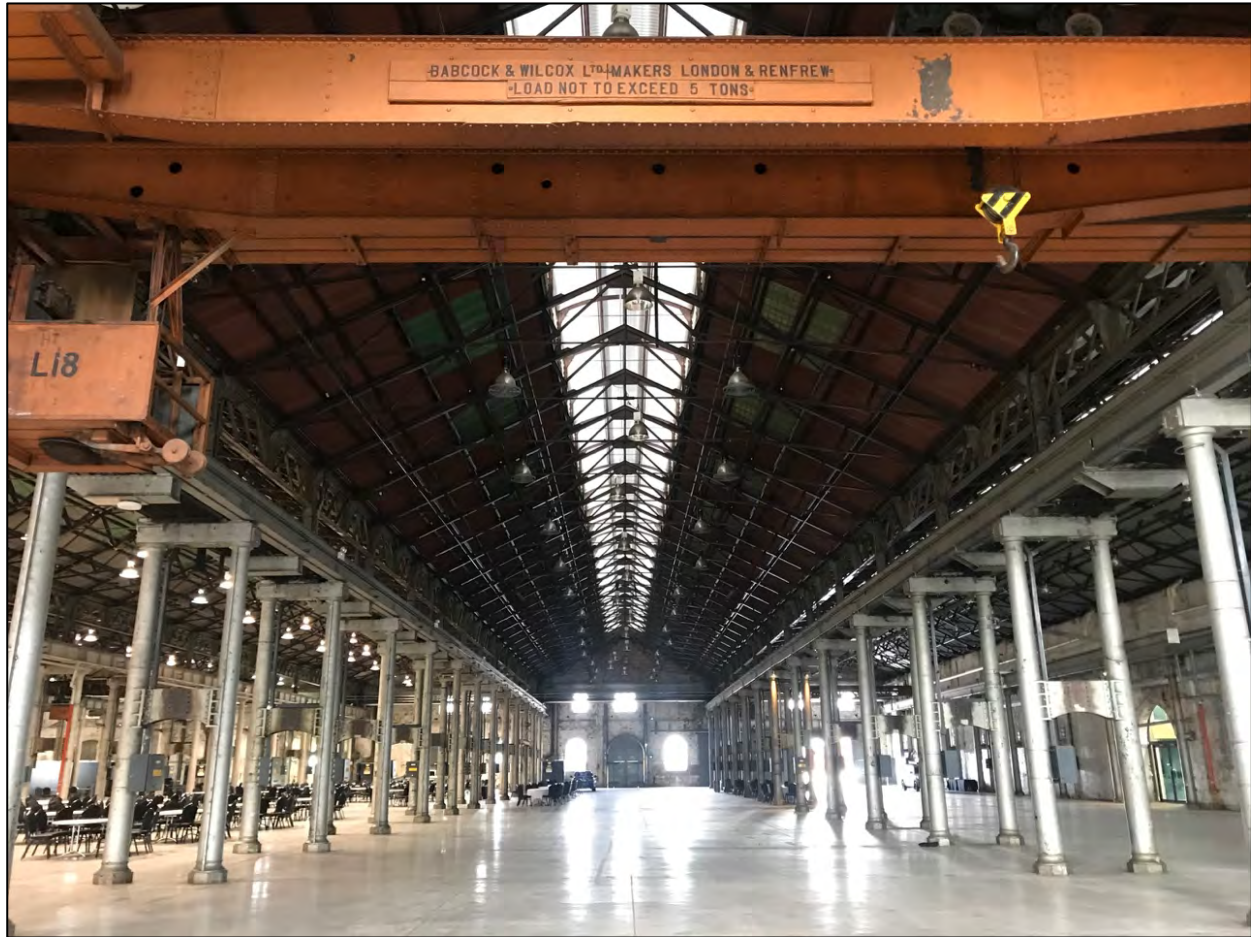
FIGURE 85: EXAMPLE OF OVERHEAD CRANE IN CURRENT EXHIBITION HALL (BAYS 9–13) (SOURCE: ETHOS URBAN 2017)
