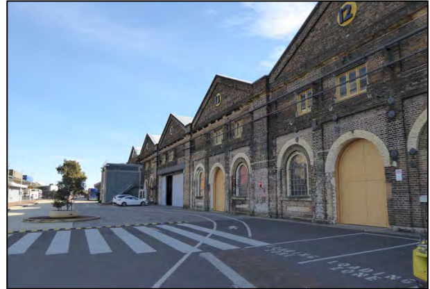
FIGURE 10: FRONT FAÇADE OF LOCOMOTIVE WORKSHOP, BAYS 12 TO 16 [NOW BAYS 11 TO 15] (SOURCE: CURIO 2016)
