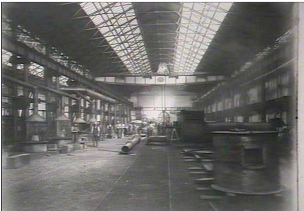
FIGURE 57: INTERIOR WORKSHOPS DURING ERW FUNCTION, VIEW TO HERITAGE TRUSSES AND ROOF SKYLIGHTS, DATE UNKNOWN (SOURCE: STATE LIBRARY OF NSW)
