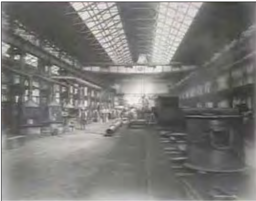
FIGURE 5: INTERIOR OF THE LOCOMOTIVE WORKSHOPS, DATE UNKNOWN. (SOURCE: GOVERNMENT PRINTING OFFICE COLLECTION, STATE LIBRARY OF NSW)
