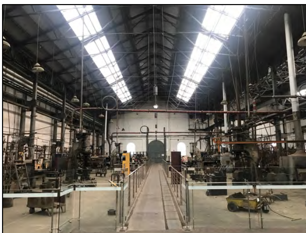
FIGURE 11: ROOF IN BAY 2, NORTH. (SOURCE: ETHOS URBAN 2016)
