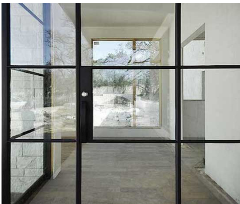
Glass infill to new external openings
