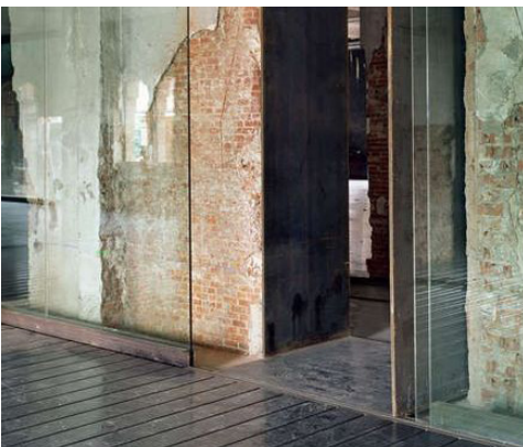
Low iron glass in front of heritage wall
