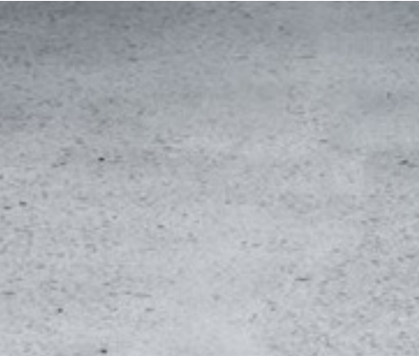
Honed concrete finish to common areas floors, Bays 1-7 ground floor.
