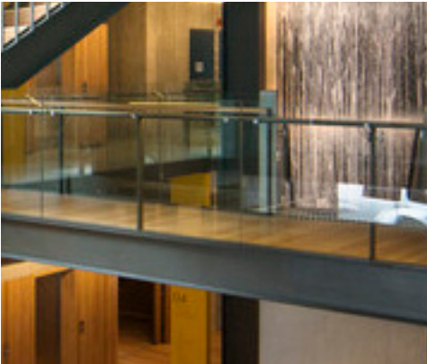
Glass Balustrade to stairs and upper floor levels to future detail bays 1-4A and 15.
