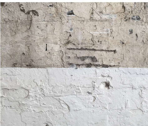
Existing painted brick wall patina conserved
