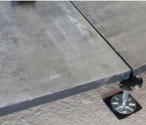
Honed concrete access tiles to central circulation within commercial tenancy, Bays 8-13 ground floor.
