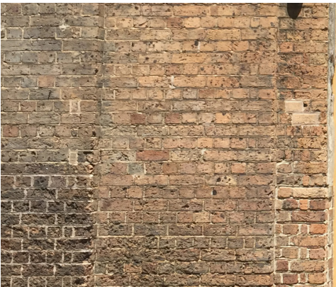
Existing heritage brick facade retained
