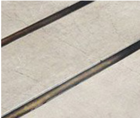
Train rack metal inlay interpretation. Runs east to west along central circulation zone in Bays 1-13
