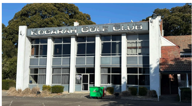
Existing Kogarah Golf Club House facing west
