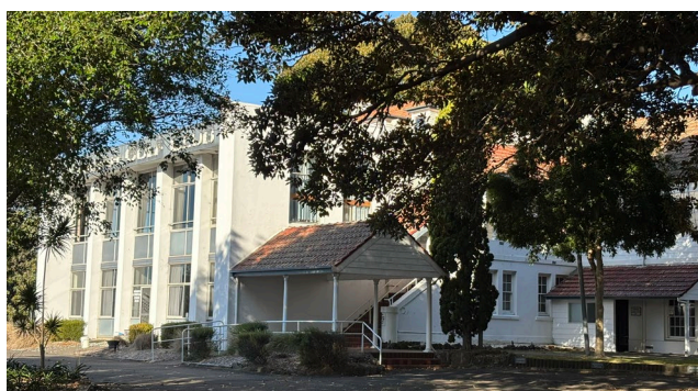
Existing Kogarah Golf Club House facing south
