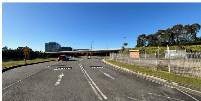
Existing Kogarah Golf Club Entrance facing south
