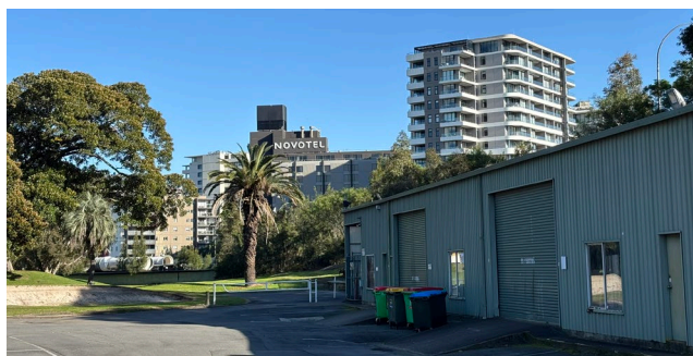
Existing Kogarah Golf Club car park facing west
