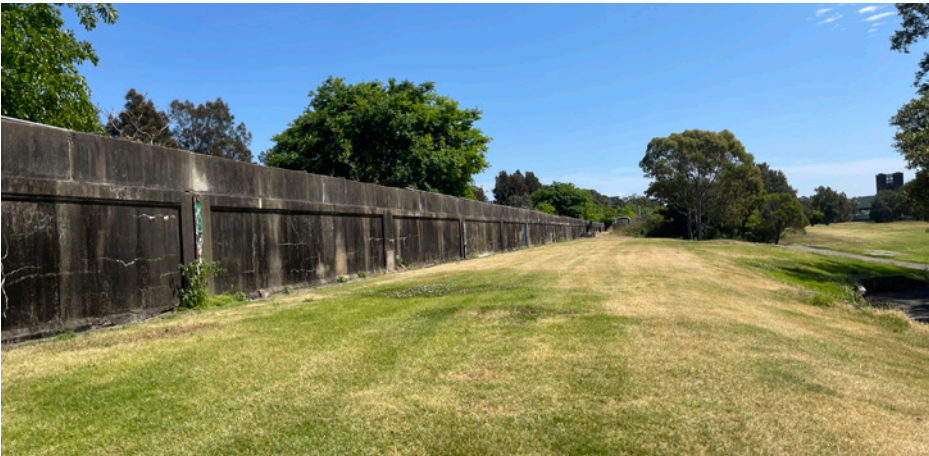
3. SWSOOS infrastructure bounding southern site (Moir 08/10/25)
