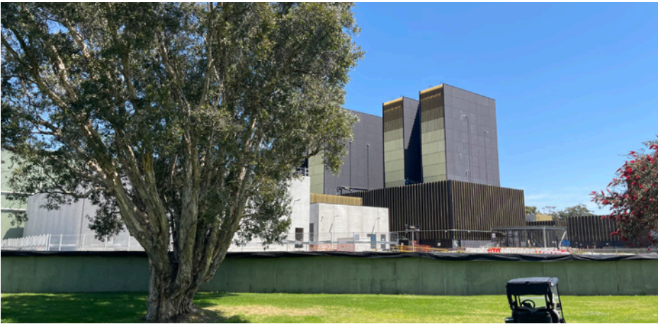
1. Back of building view from site (Moir 08/10/25)
