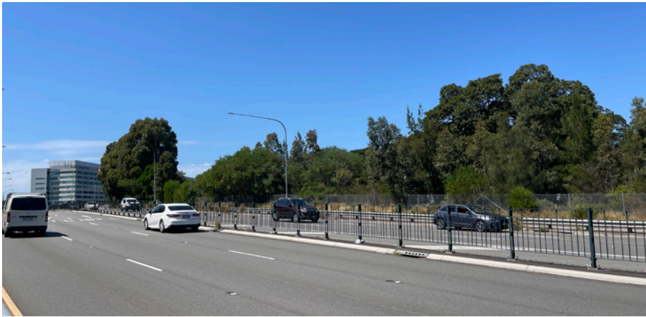
2. Road infrastructure (Moir 08/10/25)
