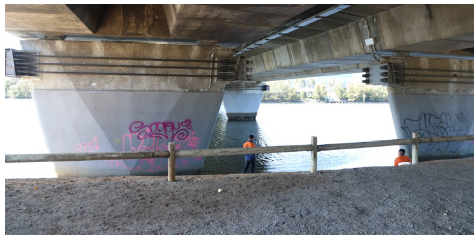
3. Under bridge (Moir 17/09/25)
