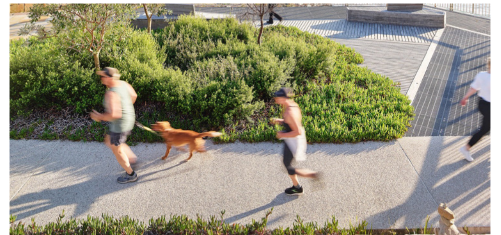
Shared path with aggregate and broom finish
