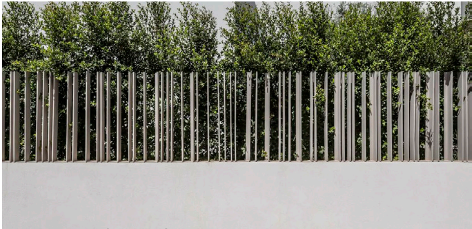
Wall and palisade fencing defining boundaries
