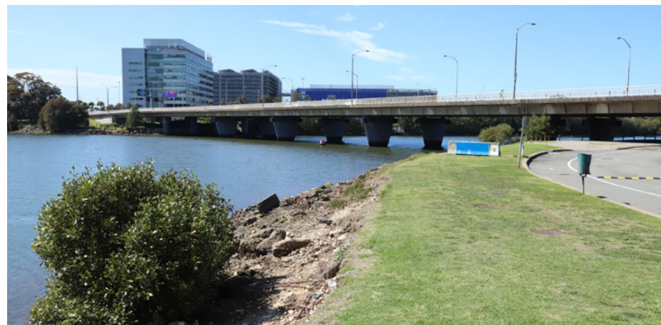
1. Giovanni Brunetti Bridge (Moir 17/09/25)
