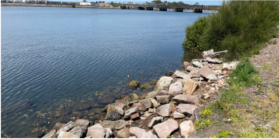
4. Southern edge condition (Moir 08/10/25)
