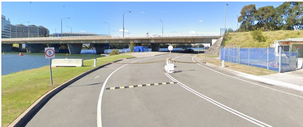
Figure 18 Existing Kogarah Golf Club access
