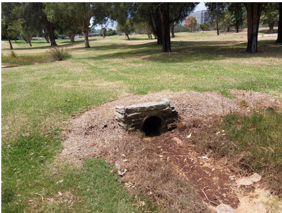
Photo 2 Small culvert located along drainage line
