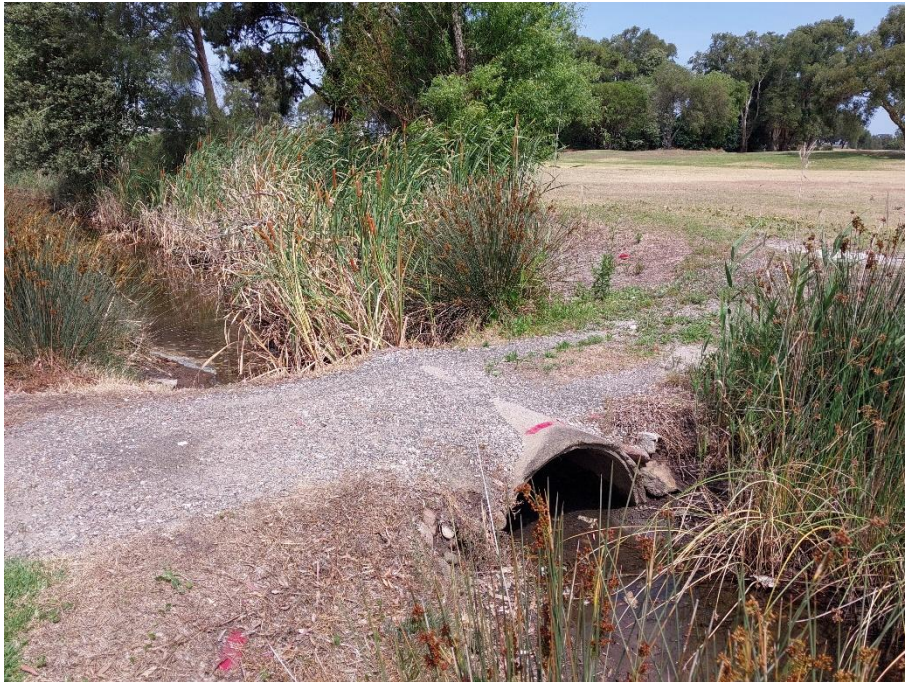
Photo 2 Small culvert located along drainage line
