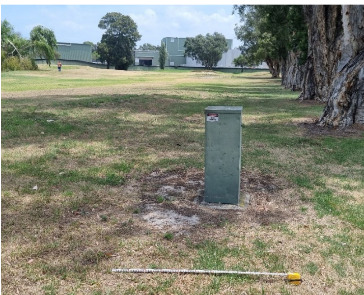
Photo 21 Subsurface electricity utilities services, facing west
