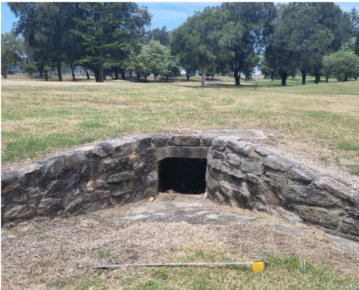
Photo 20 An example of one of an artificial water way that has been constructed and modified since at least the 1940s, facing south
