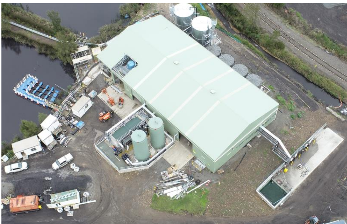
Photo 4: External of WTP shed, (right of frame) chemical unloading area and salt pit, new tanks at rear of shed
