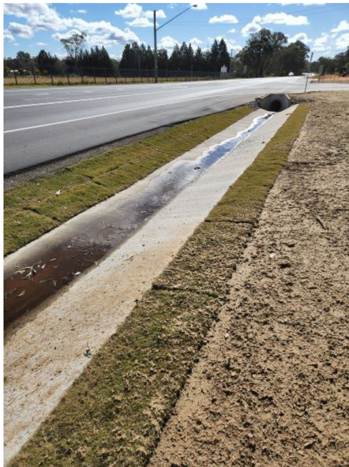
Photo 4 - Concrete and turf lined drain with temporary stabilisation applied to exposed areas
