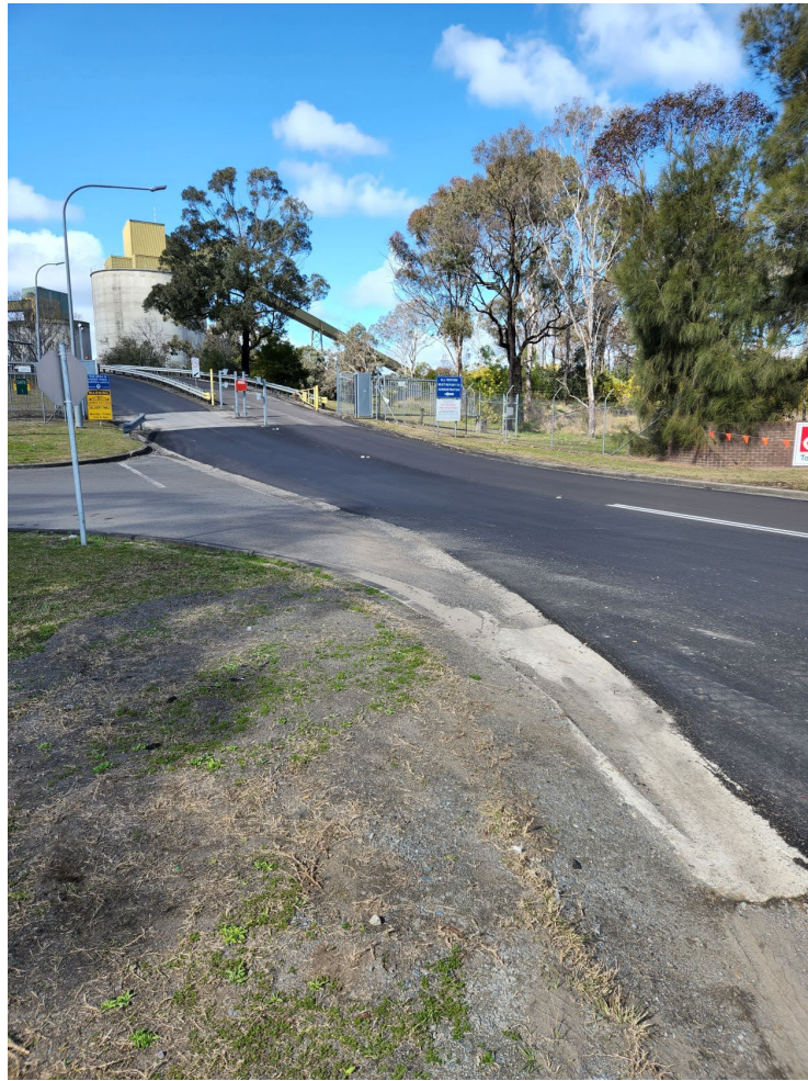
Photo 1 - Re-sealed mine access road with concrete drains
