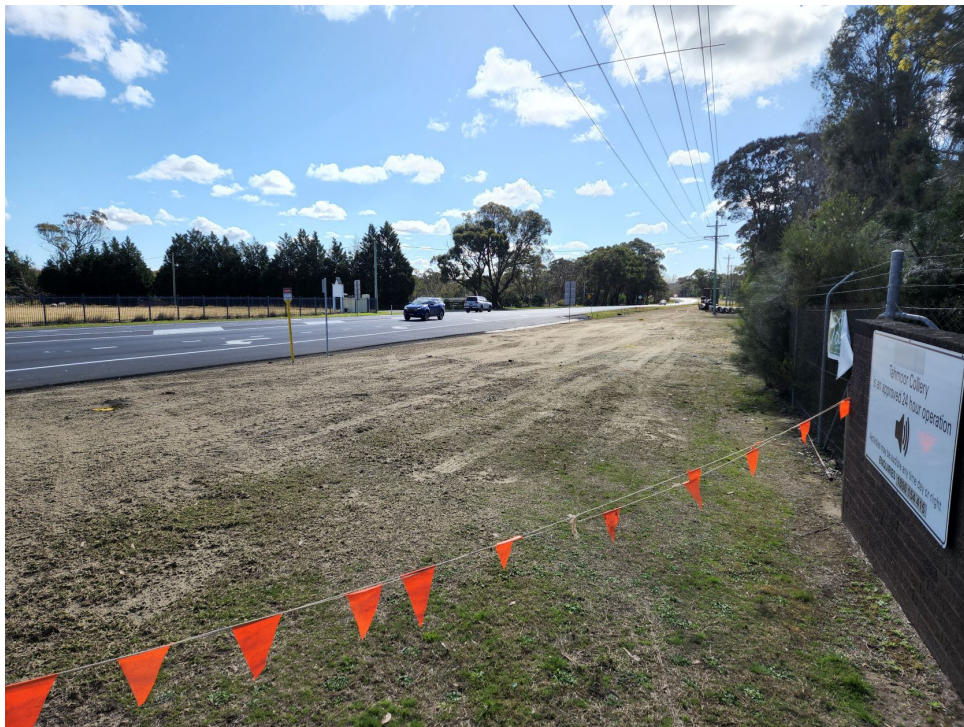
Photo 2 - Temporary stabilisation applied to exposed areas
