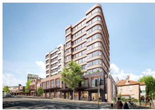
View looking north from Pacific Highway
